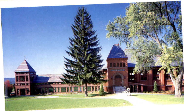
Among the Northfield School's casually scattered buildings (partial campus plan opposite), the new Dolben Library gains prominence—and stylistic precedent—from its linkage with a turn-of-the-century gymnasium recently converted to a student center (above).
