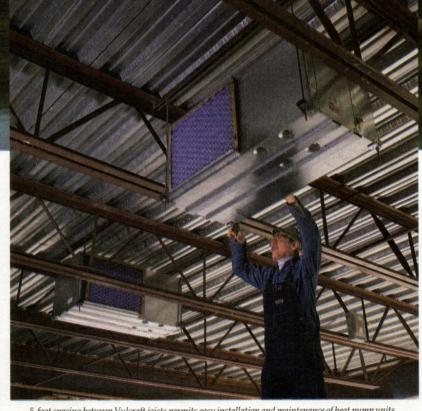
5-foot spacing between Vulcraft joists permits easy installation and maintenance of heat pump units.
