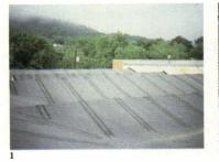
Single-ply systems are most often characterized by their method of attachment: mechanical (figs. 1, 2, 6), ballasted (fig. 3), and fully adhered. Of the two mechanical attachment configurations linear (figs. 1 and 2) and spot (fig. 6)—linear more evenly
