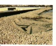
distributes stresses caused by wind uplift. The nonpenetrating attachment in fig. 6 shows the membrane movement caused by the wind, which can result in seam failure (fig. 4). Wind uplift can also redistribute ballast (fig. 5), leading to roof failure.
