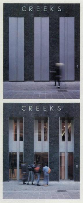
When closed, Creeks's bi-fold aluminum shutters make the facade an impenetrable plane (top). When opened, the glass doors provide an enticing glimpse into the cottoncandy-colored interior (bottom).
