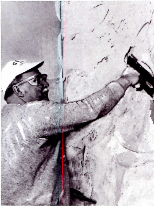
BEST WAY. Portland cement mortar over lath was great when labor costs and time delays were acceptable.
