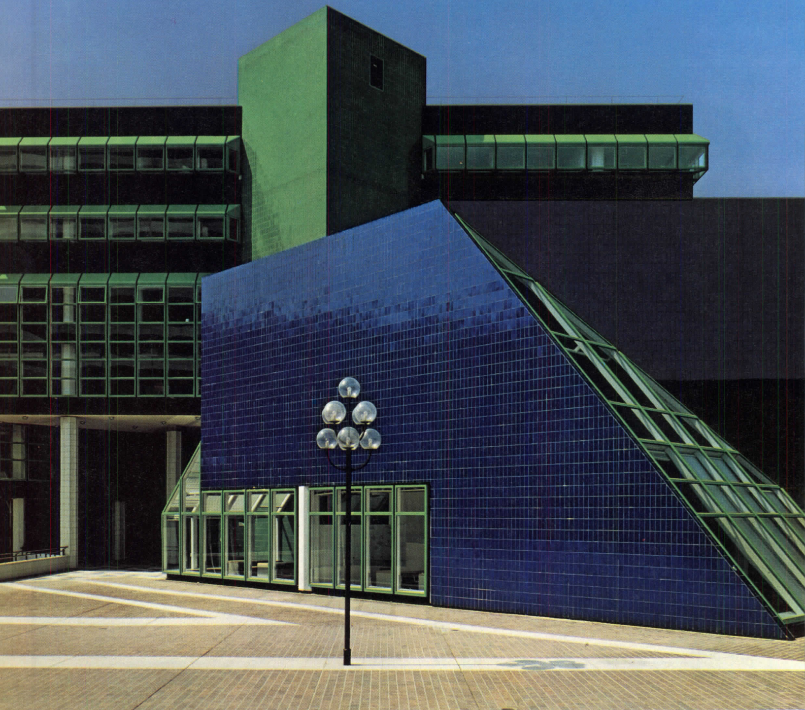
Cergy Pontoise Hotel, near Paris, clad in Monocolor #144 Intensive Blue and #143 Intensive Green. (Thin-set latex mortar on precast concrete. Architects: Claude Vasconi and Georges Pencreach.
