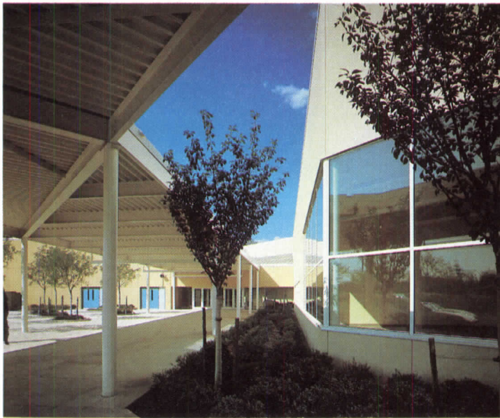
The Bleshman School is one of the first ever designed specifically for the multiple-handicapped rather than adapted from conventional facilities. Public bond issues funded the $3-million project, a concrete block structure with an insulating layer of rigid styrene and a synthetic plaster finish. The entry porch (above), open courtyards, and nature paths extend school activities outdoors.
