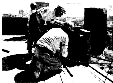
Part of Curtain Wall Support System galvanized with Z.R.C., IDS Center, Minneapolis—Also used on Curtain Wall Mullions, Republic Bank Tower, Dallas.
