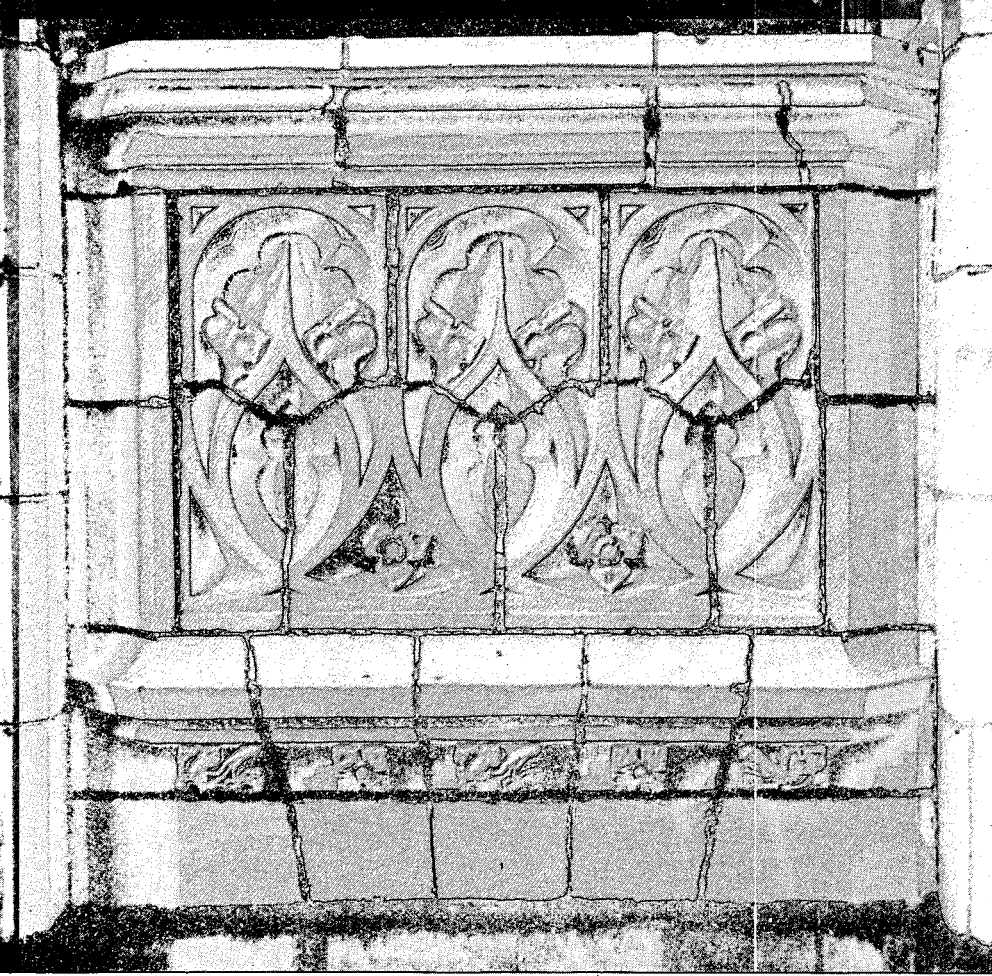
Concrete masonry replacements for damaged spandrel panels were cast in molds struck from the original terra cotta. Two-step casting allowed replication of integral background color. Below: The complex curves of the haunches under the building's elaborate projecting canopies were matched in polymer concrete poured in place into fiberglass molds formed on similar haunches. Damaged pendants that could not be repaired by other means were strapped into wire baskets (bottom right).
