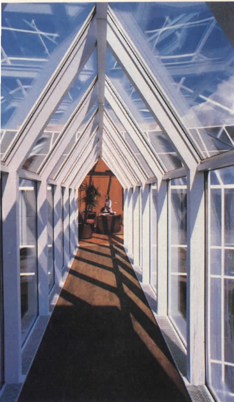
A steel-framed pedestrian bridge (above) connects the free-standing elevator tower to the garage, ground, and third levels. The concave facade (left) emphasizes the entrance and preserves as much of the landscape as possible.
