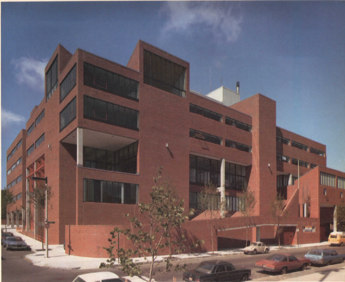
Peter Vanderwarker photos except where noted
