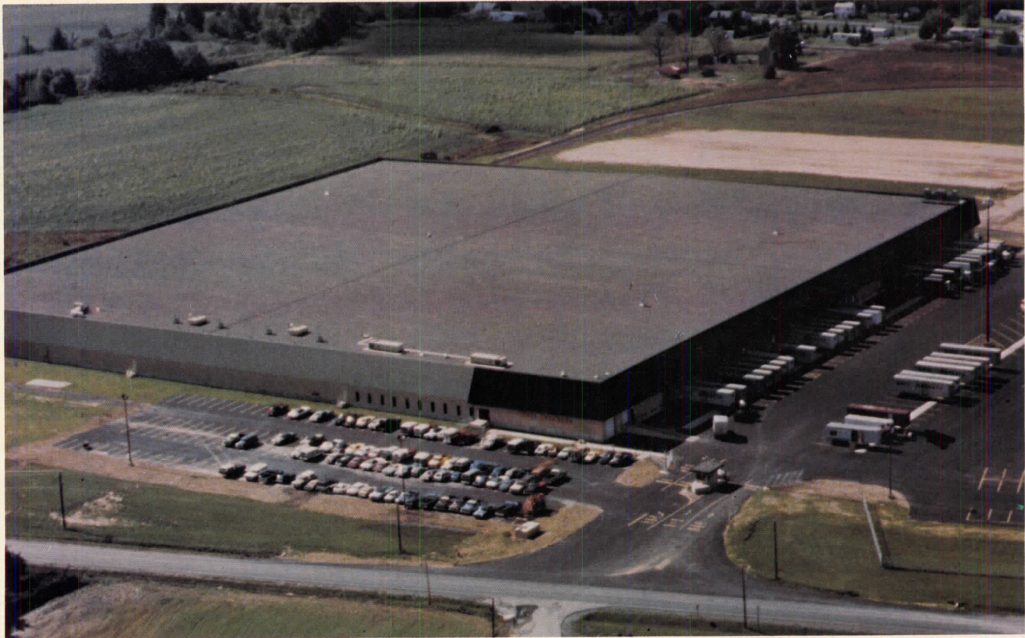
Aerial view of the Carlisle roof on the new Milton, Pennsylvania Distribution Center built by Weis Markets, Inc.
