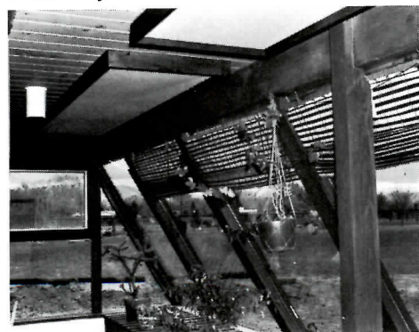
Panels above greenhouse extension
