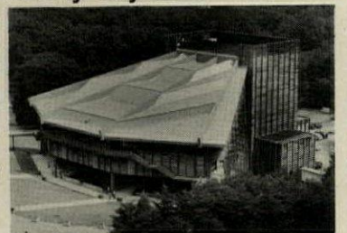
New roof on Filene Center at Wolf Trap Farm Park, Va., 1974. Overly batten roof stopped leaks.
