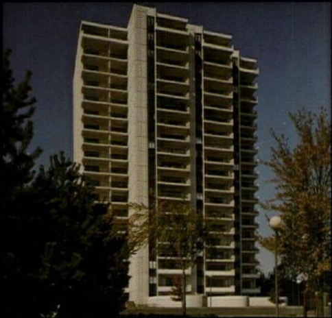
AMERICAN PLAZA TOWERS PORTLAND, OREGON
