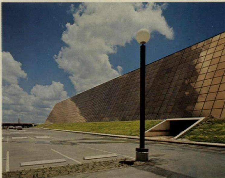
Architect: Neuhaus + Taylor, San Antonio, Texas Glazing Contractor: Samuels Glass Co., San Antonio, Texas
