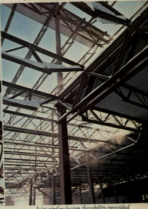
Joist girder design flexibility provided for a wide range of load support, from normal roof loads to heavy mechanical equipment loads.
