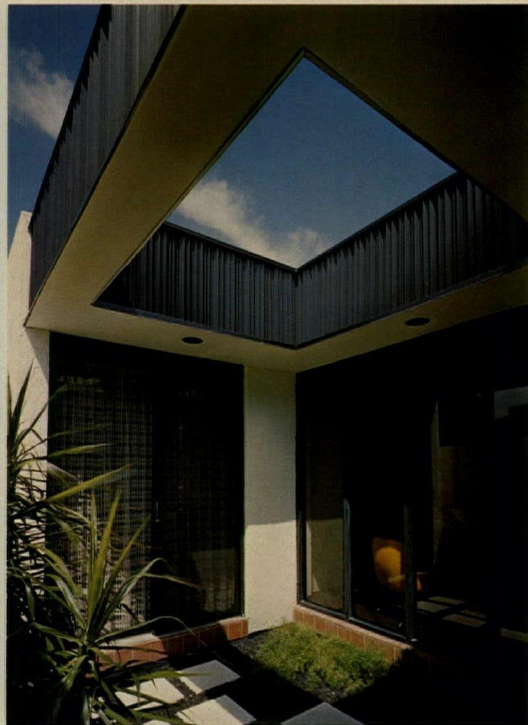
Project: Professional Building for Stebbins & Scott, Fort Pierce, Florida Architect: Stebbins & Scott, A.I.A. Fabricator/Installer: Construction Specialties, Inc.
