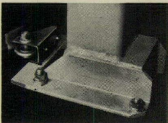
6" x 6" steel support posts.
