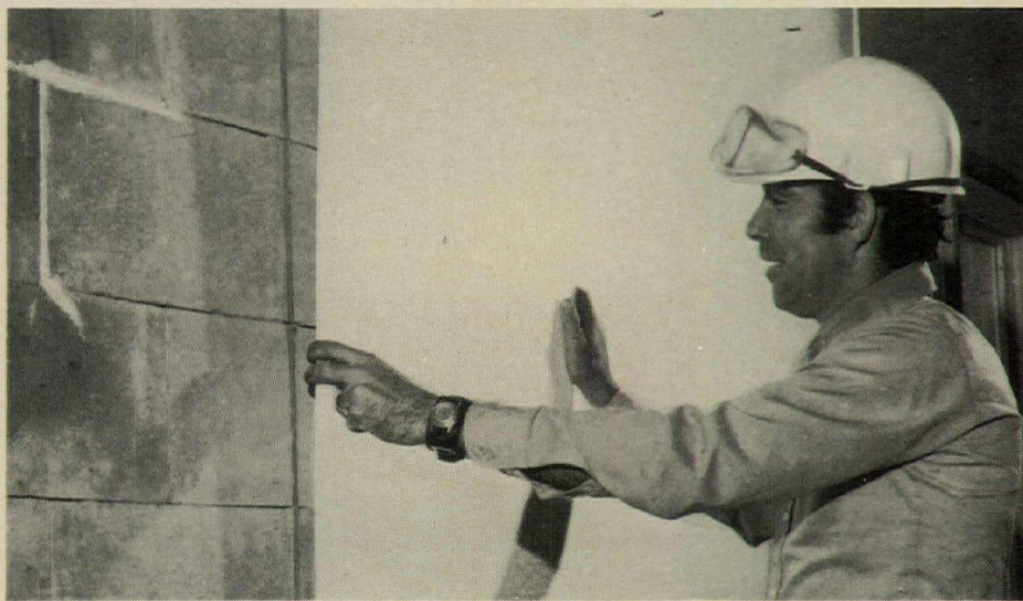
Position ZONOLITE Styrene Foam.
