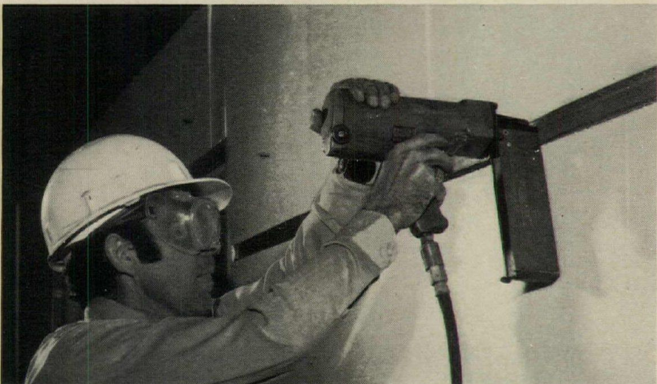
Nail through Foam to masonry.
