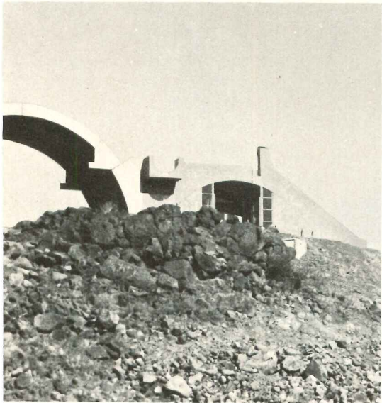
The bright coloring on the underside of the Vault (above, left and right) was painted onto dried river silt, which had been previously layered over the wood formwork. After concrete is poured over this painted silt and allowed to set, the forms are removed, the excess silt washed off with water, and the color remains in the concrete. This "silt casting" technique is used throughout Arcosanti.
