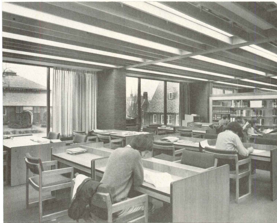
Open board ceilings conceal the mechanical equipment and carry lights and acoustic material.
