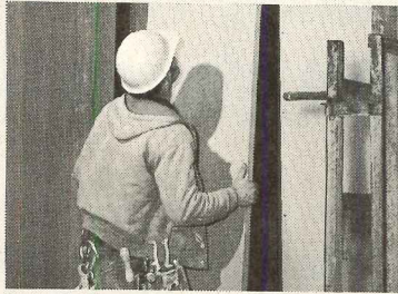
2. Installing core panel.
