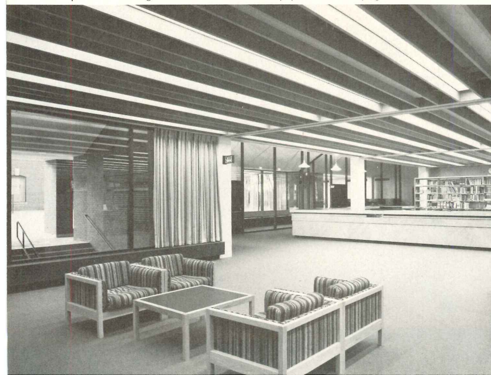
Open board ceilings conceal the mechanical equipment and carry lights and acoustic material.
