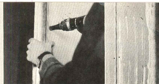
3. Attaching core to T-spline.
