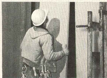
2. Installing core panel.
