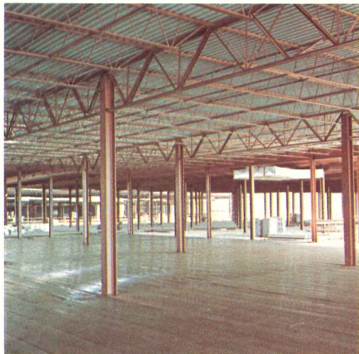
Joist girders need fewer foundations and columns. Which means less work for you and larger bay areas for your clients.
