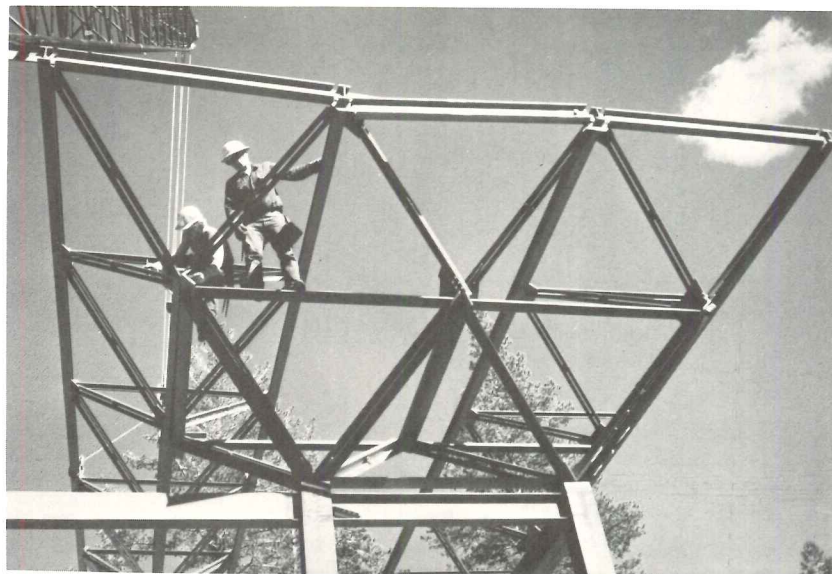
There are four space trusses (as the one above) comprising the roof structure for the lodge. All connections between the column frames, the support trusses, and the main-span trusses are made in the field using high-strength bolts. The 8-ft gap between top chords of the main trusses is spanned by 16-gage corrugated metal decking, 3-in. deep.
