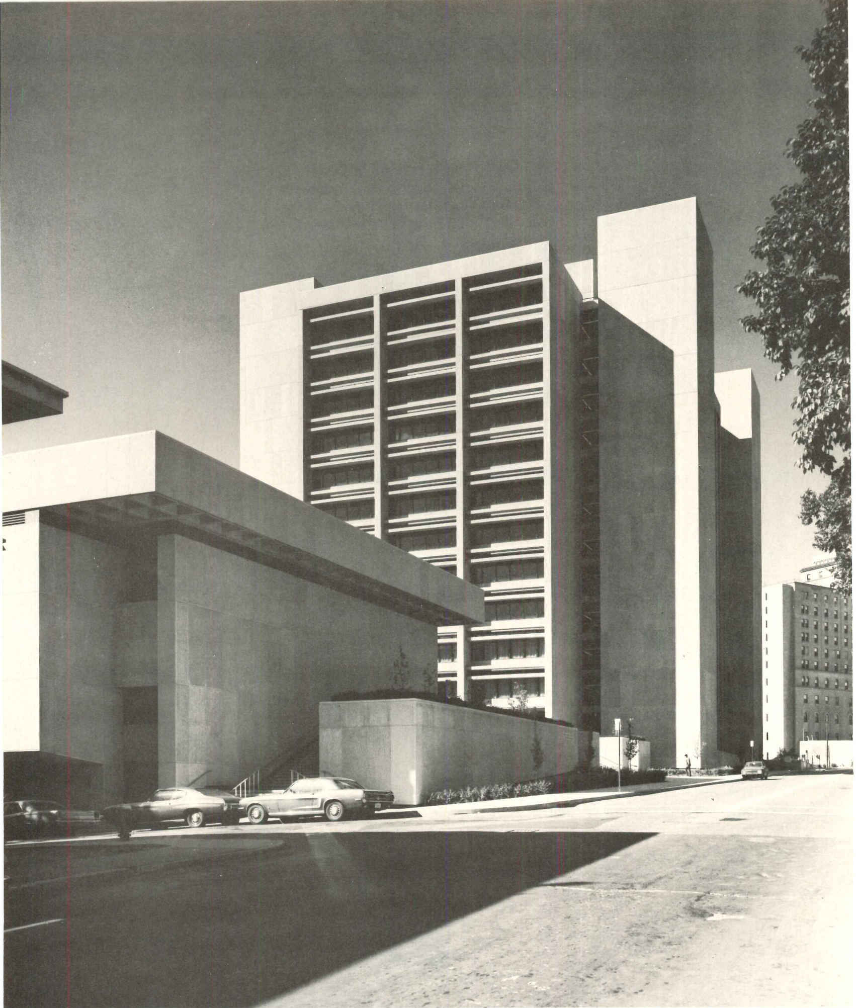
UNIVERSITY OF PITTSBURGH SCHOOL OF ENGINEERING (Michael L. Benedum Hall). ARCHITECTS: Deeter Ritchey Sippel Associates. BUILDER: General State Authority, Commonwealth of Pennsylvania. Dover Elevators installed by Marshall Elevator Co.
