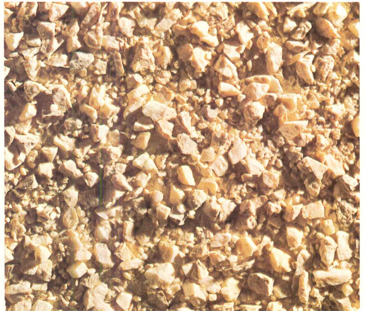
2. The stone wall.
