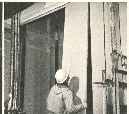
2. Installing core panel.
