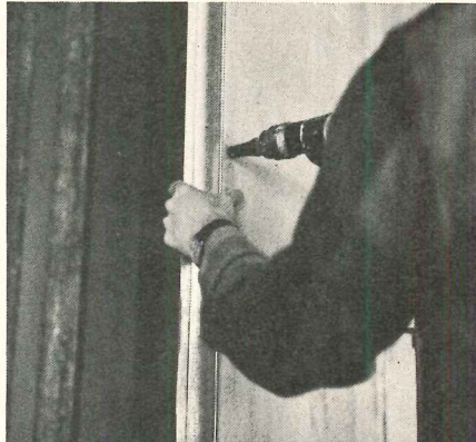
3. Attaching core to T-spline.
