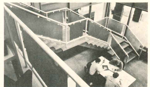
PIPE RAILING SYSTEM / Components of this aluminum system are connected by tubular rivets and machine screws at intersections, and by epoxy adhesive at splice joints. ■ Julius Blum & Co., Carlstadt, N.J.
