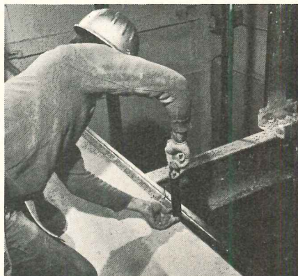
1. Installing floor track.
