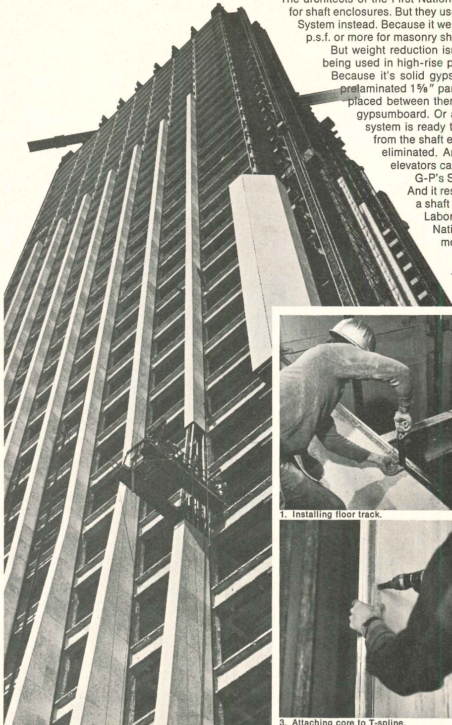
3. Attaching core to T-spline.
