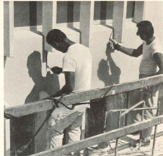
F. final touch up and cleaning of joints
