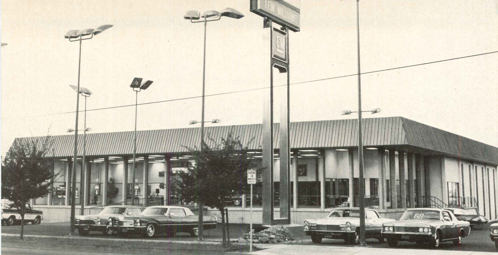
Lew Williams Cadillac, in Portland, Oregon, uses a Lennox roof mounted, gas-electric, single package air conditioner to heat and cool this showroom and office.
