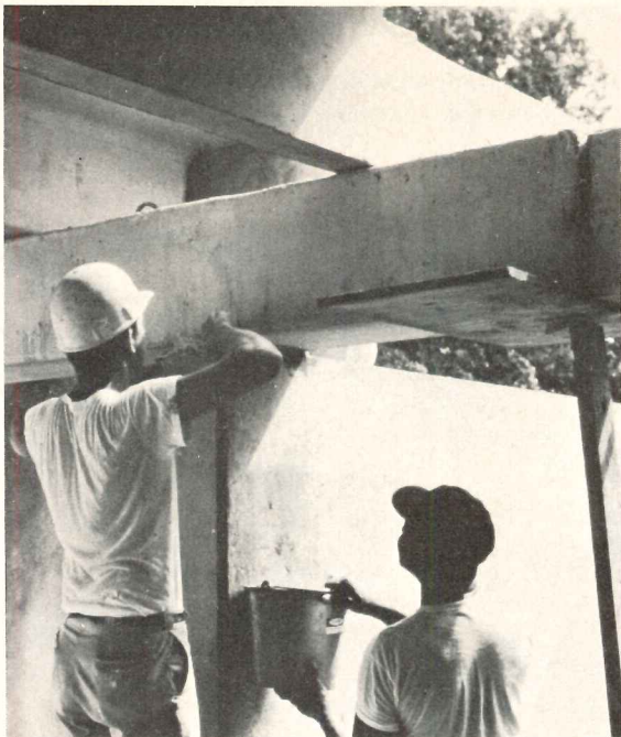
7. Placing epoxy grout between beam and core
