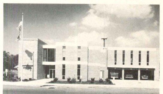
Manchester City Hill (above) is one of several municipal buildings designed by the firm in the Tennessee region. It combines municipal administration, fire station and police department. Such combinations of function are common in the medium cities of Tennessee which usually face stringent budgets.
