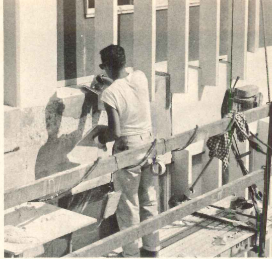
B. leveling the sills
