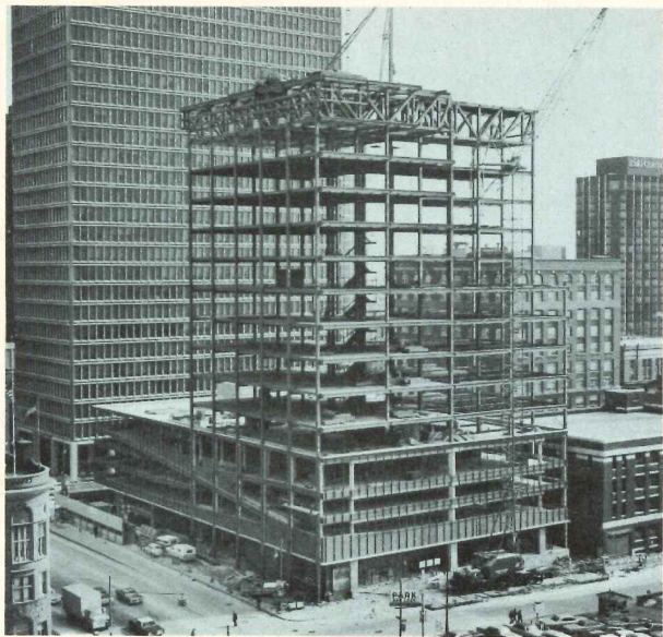
This framing system shows how suspended intermediate columns help provide maximum column-free floor space in garage and first floor of the tower. Truss support is carried by the 12 exterior and 6 interior load-bearing columns.
