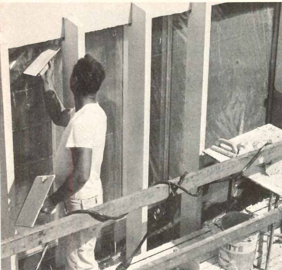
D. vertical and overhead troweling
