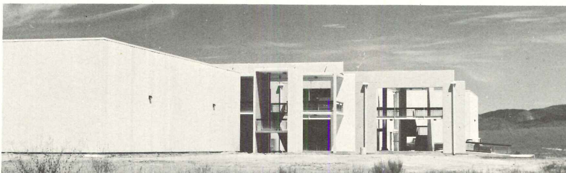
Carson City High School , Carson City, Nevada, Selden and Stewart, architects with Caudill Rowlett Scott is phase I of a "school community," focused on a "main street." Circulation is through pedestrian galleries joined by bridges. The structure is planned to be
