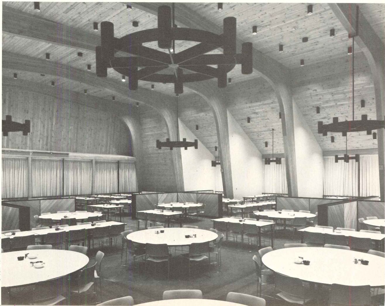
The dining hall (right and below)—another key building—shares its architectural vocabulary with the student activity building and the gym. Wood bent construction has been used to ease footing loads because of poor bearing.
