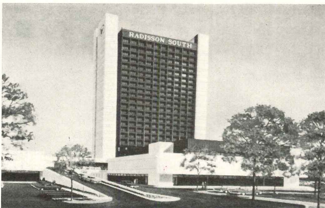
RADISSON SOUTH HOTEL, Minneapolis, Minn. Owner: Radisson Management Association Architect: The Cerny Associates, Inc. Structural Engineers: Intertec, Inc., and The Cerny Associates, Inc. General Contractor: Earnest M. Ganley Construction Co. Fabricator: Paper, Calmenson & Co. Erector: L. H. Sowles Co.
