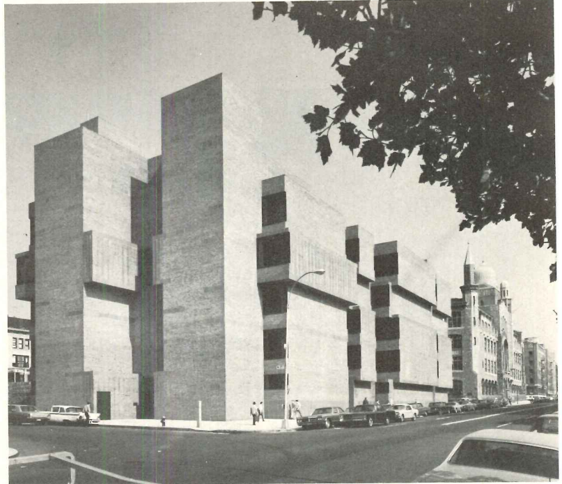
Yeshiva University Library , New York City, Armand Bartos and Associates, architects, contains two libraries, a museum, a music collection, a microfilm center, and an archives collection. Separate entrances are provided for visitors and students. Structure is of concrete with brick infill.
