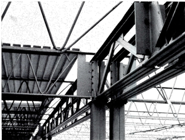
Macomber V-LOK connectors at the column lines . . .
