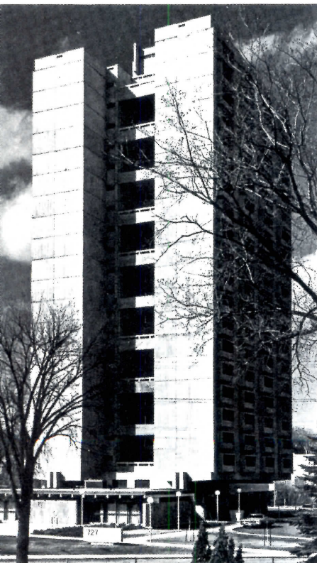
727 Front Avenue , St. Paul, Minn., Freerks, Sperl, Flynn, architects, St. Paul, high-rise apartments of exposed reinforced concrete are oriented to face the two major views from the site.
