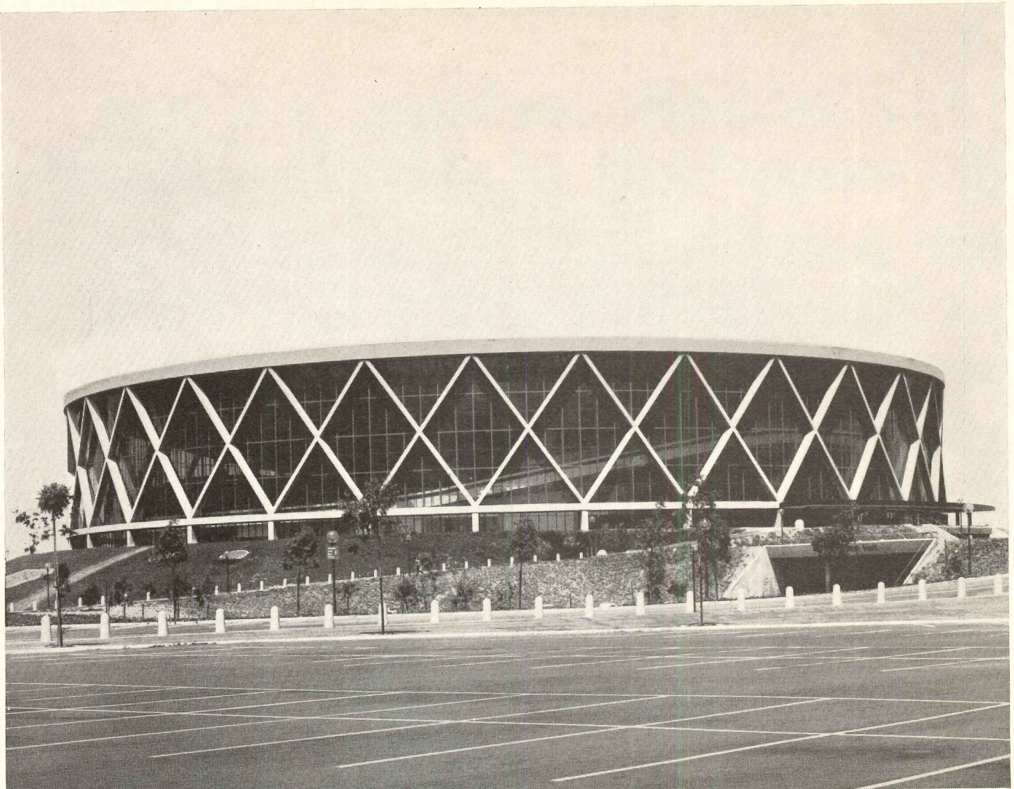
Oakland-Alameda County Coliseum Complex Arena Building Architects/Engineers: Skidmore, Owings & Merrill, San Francisco
