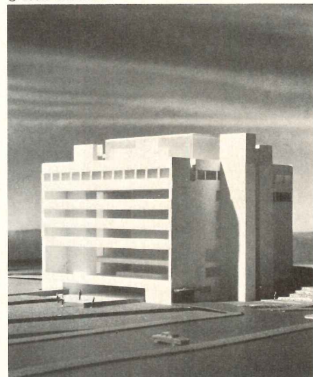
St. John's University School of Law , Jamaica, N.Y., Carson, Lundin & Shaw, architects adheres to a five-foot square module, and is square in plan. Arrangement of glass openings was determined totally by function. Stair and restroom towers flank a central axial corridor. Brick facades and upper story articulations are meant to harmonize with nearby buildings.
