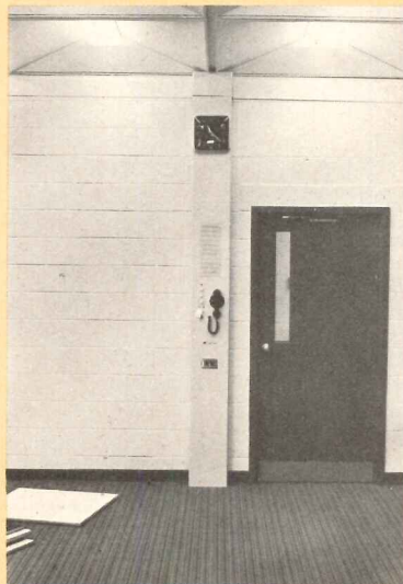
Heart of the system is the ceiling distribution box which feeds power to lights and to receptacles, sound signals to speakers and intercom set on service column, and ties fire detectors and manual fire stations to the communications control center. Fire alarm is simulated siren over loudspeakers.
