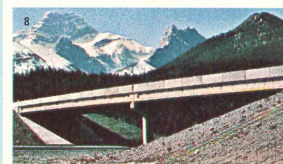
8. PRECAST PRESTRESSED GIRDER BRIDGE 9. TENDONS IN PLACE FOR POST-TENSIONED SLAB
