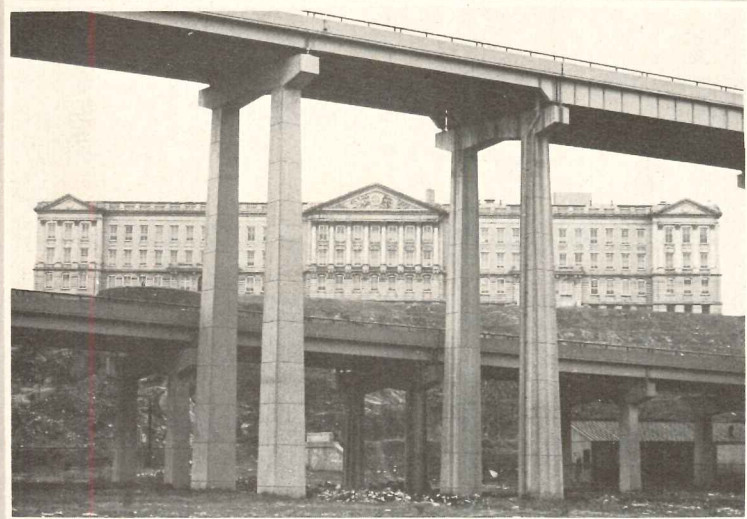
NEW JERSEY TURNPIKE/JERSEY CITY HIGH SCHOOL
