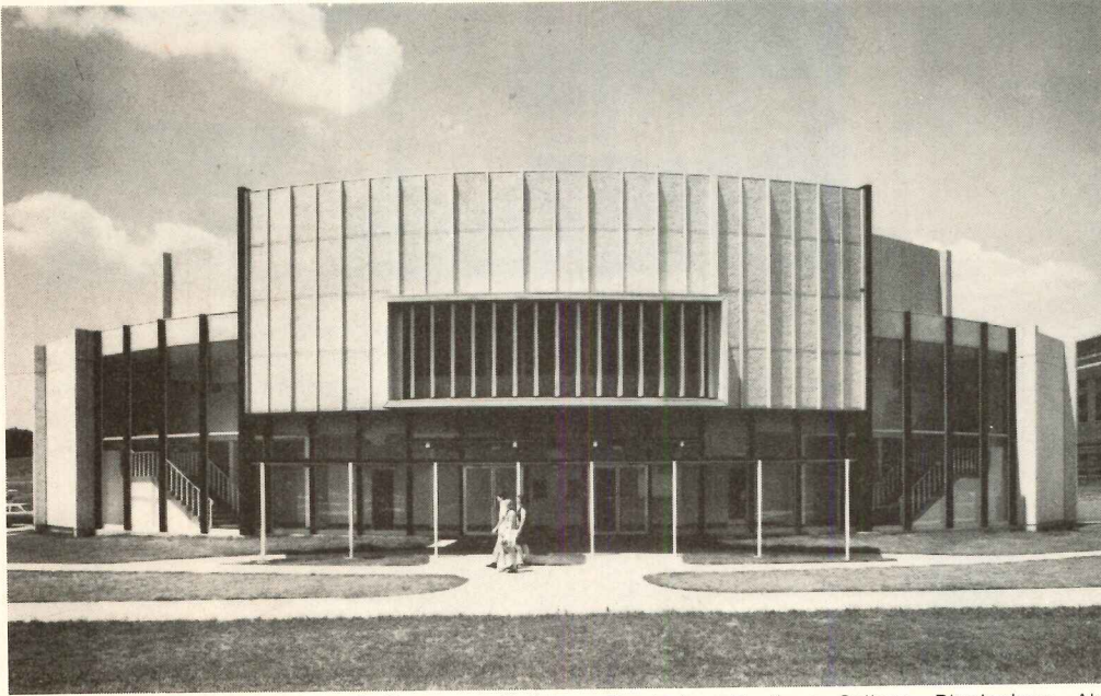
Theater and Classroom Building, Birmingham-Southern College, Birmingham, Ala. Architects: Warren, Knight & Davis. Theater Consultant: Dr. Arnold Powell. General Contractor: Brice Building Company, Inc. Dover Stage Lift installed by Dover Elevator Co., Atlanta.
