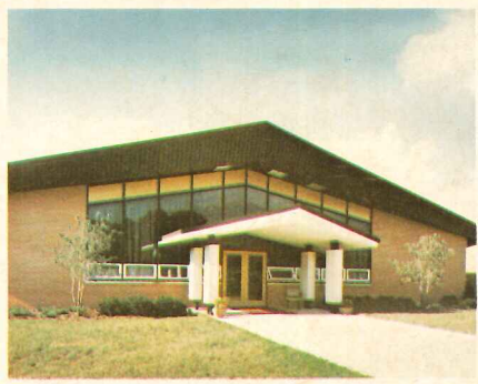
ARCHITECTURAL ENTRANCE SYSTEMS FORM ATTRACTIVE FRONT . . .
