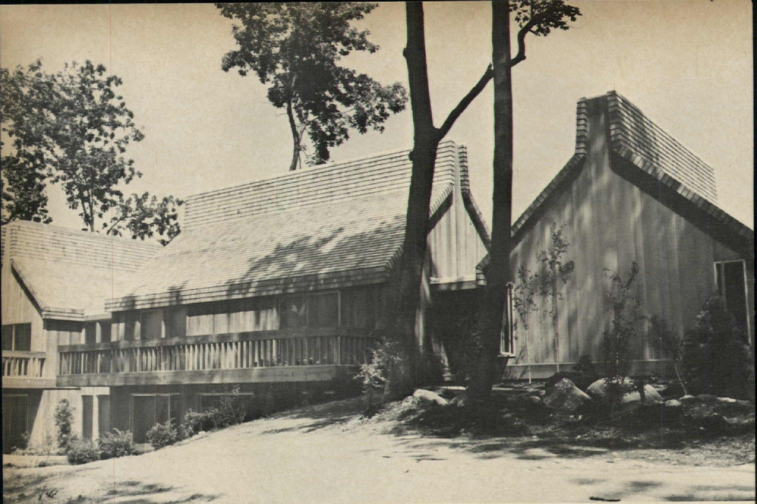
Architect: Delnoce Whitney Goubert Builder: Frank H. Taylor and Son, Inc.
