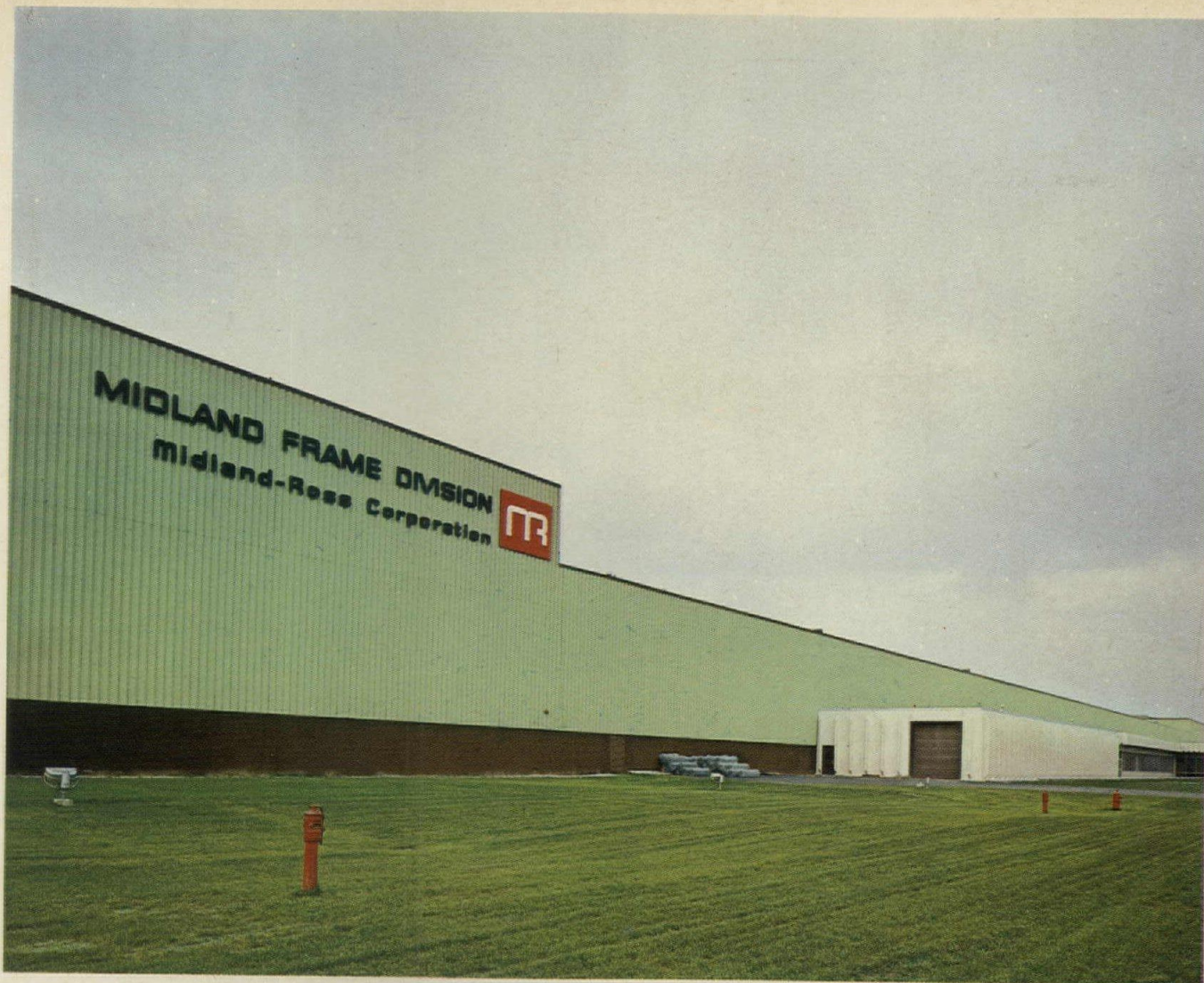
Frame Division Plant. Owner: Midland-Ross Corporation, Maumee, Ohio. Contractors: Lathrop Company, Toledo, Ohio. Engineers and Architects: Rossi & Nickerson, Toledo, Ohio. Finish: Metal walls finished with Fluropon† made with Kynar 500.
