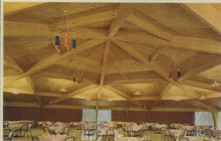
Architects: Marshall M. Burton & Associates
