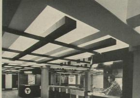
aided through new lighting. Glare-free fixtures light both ceiling and floor; they are heavily constructed to withstand vandalism. Special lighting accents graphics along platform and between tracks. Downlights demark the turnstile area.
