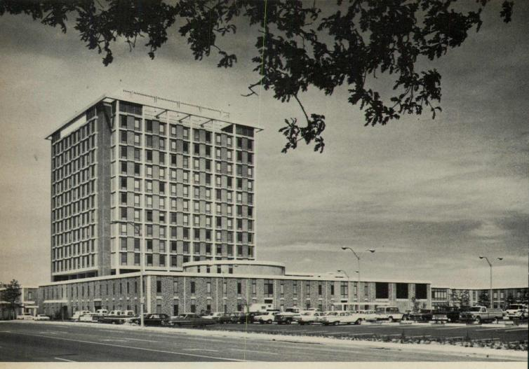
ABOVE—Veterans Administration Hospital, Memphis. Architects: A. L. Aydelott and Associates. General Contractor: Henry C. Beck Co. Seven Dover Gearless Elevators with Computamatic group supervisory control; 4000/5000 lbs. capacities; 500 FPM. Three Dover Oildraulic Elevators; 5000/6000 lbs. capacities; 60 FPM. Installed by Dover Elevator Co.
