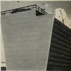
Ruberoid Corrugated Asbestos Sheets are an economical, weather-proof and fire-proof construction material for industrial buildings. Resistant to corrosion, maintenance-free indefinitely!
