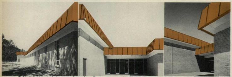
THE UNUSUAL fascia design that is also used as soffit trim, shown above from various angles, is of standing seam construction, fabricated from 25,000 lbs. of Revere 16-oz. cold rolled copper. Structure is the W. J. WOODHAM HIGH SCHOOL, Pensa-
