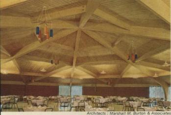
re-shrunk to full American Lumber Standard sizes, South-n Pine provides stability and precision essential to engiered construction, as in this country club. Standard grades n be utilized for cantilevered and continuous members thout special grading.
