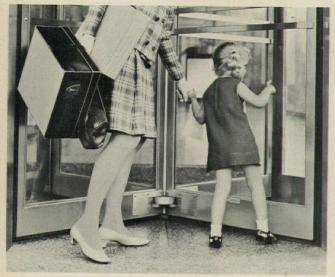
A finger, a hand, an elbow, a hip, a knee or a toe pushed gently against any part of a wing starts the door turning.
