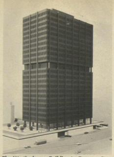
The Westinghouse Building in Gateway Center, Pittsburgh, designed by Harrison and Abramovitz and owned and operated by The Equitable Life Assurance Society of the U.S., will be a 23-story office building of steelframe construction with cellular steel floor decks. The building, which will contain 500,000 square feet, will have an all-electric system, with the heat from the lighting system utilized for needs within the building.
