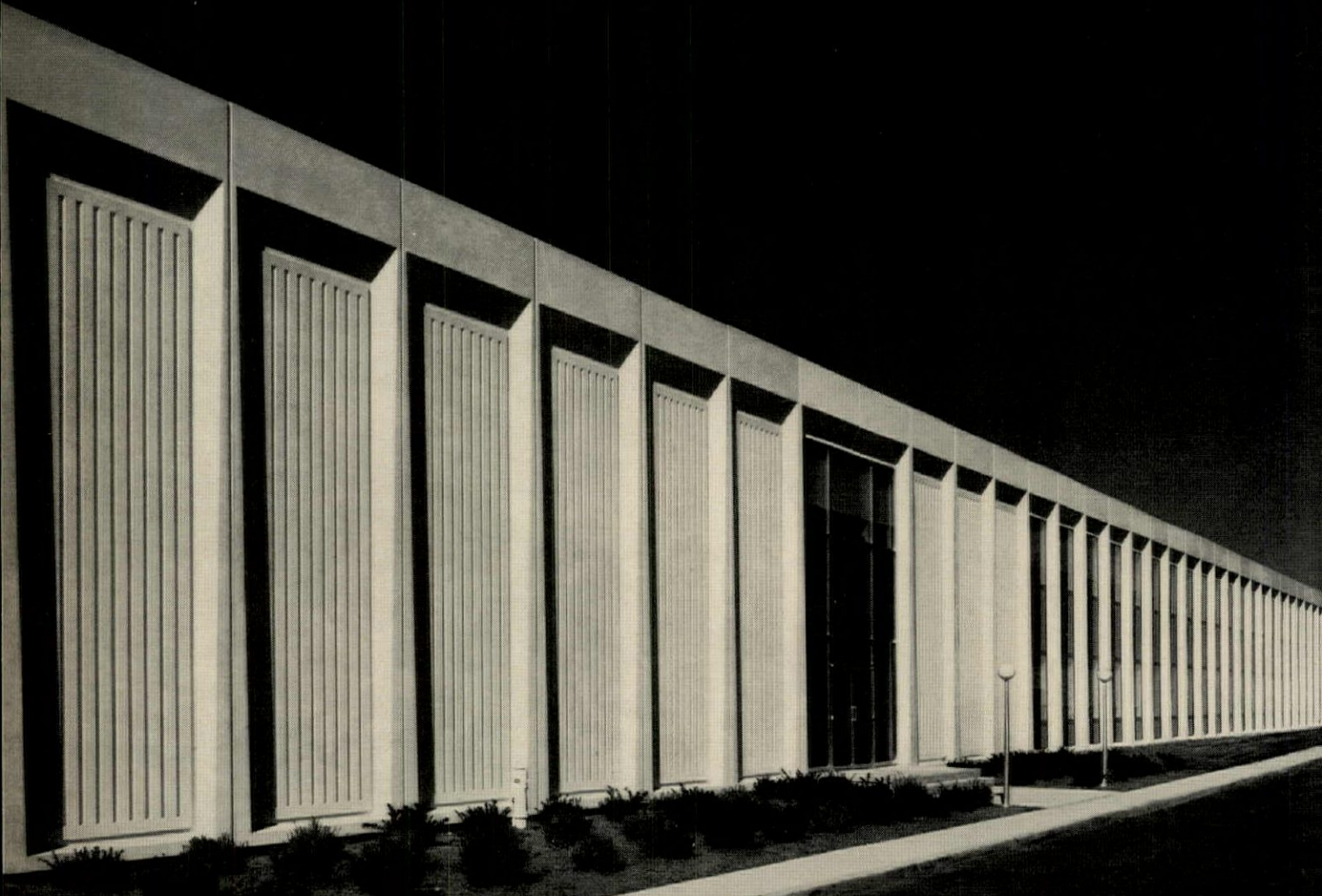
Schokbeton precast concrete curtain wall, Dell Publishing Warehouse, Pinebrook, New Jersey Architect: Frank Grad & Sons, Newark, N.J. Schokbeton by: Eastern Schokcrete Corp.
