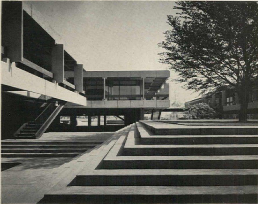
The photograph above shows the way ground levels were handled beneath and between buildings to provide semi-hidden parking and attractive spaces.
