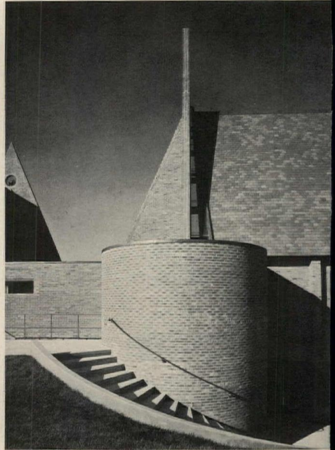
Cylinder adjoining chapel encloses interior stair.
