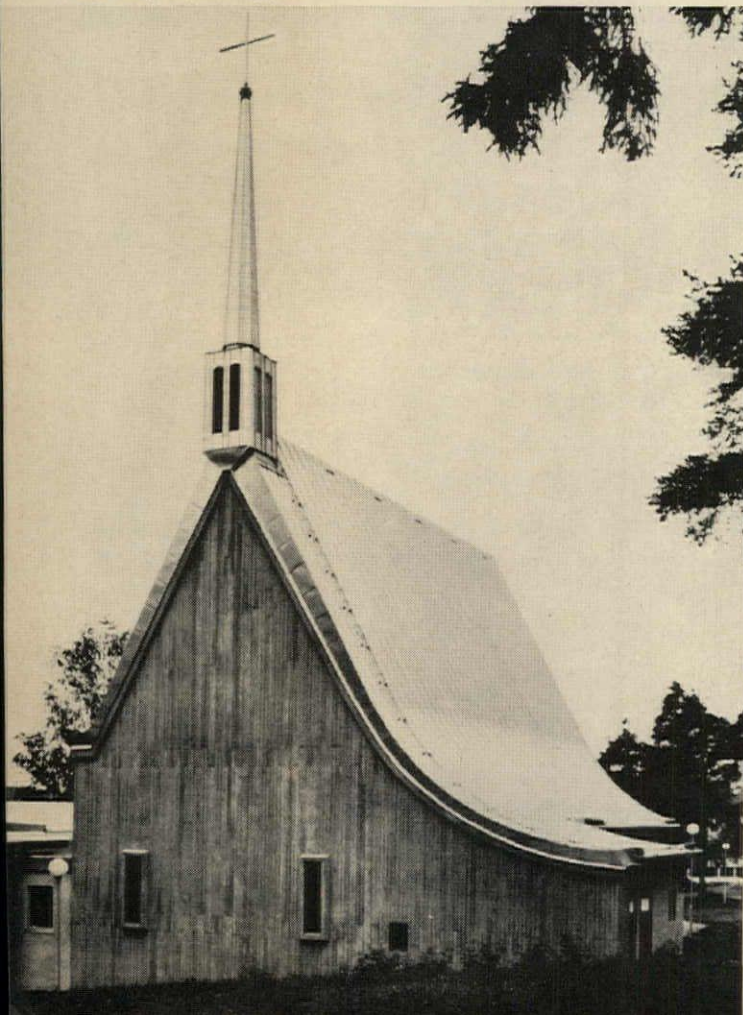
All Saints Church, Sodertalje, Sweden. Architect: Rolf Bergh, Sodertalje, Sweden. Stainless steel roof: Fagersta Bruks AB, Fagersta, Sweden and Fagersta, Inc., Chicago, Ill.
