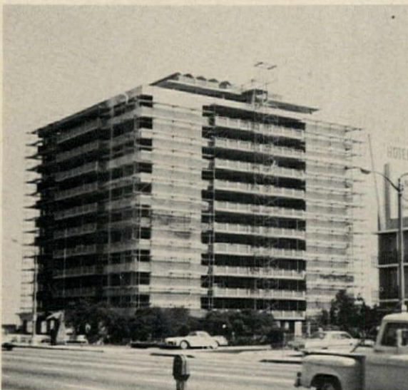
A 15-story apartment building in Long Beach, California has prestressed core and floor slabs prestressed in both directions. Post-tensioned floors serve as diaphragms to transmit wind and earthquake forces to the core. Architect, James R. Wilde.
