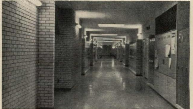
Hillyard Hil-Tex undercoater-sealer used on all corridor and classroom floors (resilient). Super Hil-Brite carnauba wax used for floor protection and easy daily maintenance.
