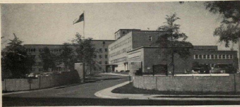
Maryland Veterans Administration Hospital
