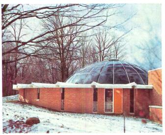
The Kalamazoo (Michigan) Nature Center is one of the latest in a growing number of dome structures, glazed with Plexiglas® acrylic plastic, constructed to provide a natural environment indoors. Light and heat control is attained through the use of transparent gray #2064 Plexiglas, one of a full range of transparent tints available to satisfy varying requirements for light transmittance, glare control and solar heat reduction.
