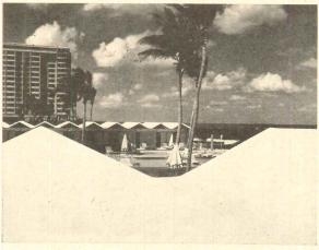
A single ply of roofing gives long-lasting whiteness to the prominent, folded-plate roof of this hotel cabana. The surface of Du Pont TEDLAR\* PVF film will remain a brilliant white, even after years of exposure. The roofing is Ruberoid T/NA 200† with TEDLAR. T/NA 200 is easily installed with conventional roofing techniques. It weighs less than conventional built-up roofing, and it can fit roofs of unusual contour and of any slope.
