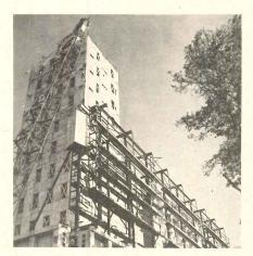
Start of truss is at the center bay with one column being erected first
