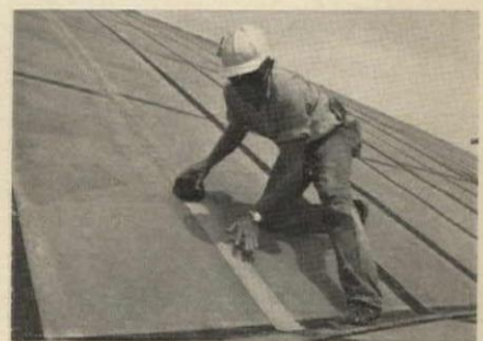
Top: Neoprene applied with pressure-fed rollers over glass roving. Above: Elastomeric tape seals joints. Below: Coating panels between skylights
