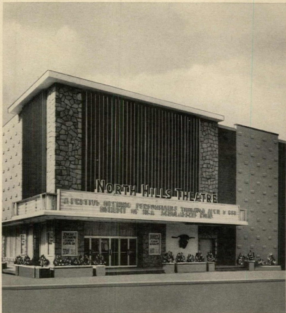
NORTH HILLS THEATRE , Pittsburgh, Pa., is air conditioned by four York "packaged" Embassy units. Owner, Stanley Warner Theatre Corporation; Architect, Drew Eberson, A.I.A.; General Contractor, Harry Dunn Company; Contractor, Marchese Refrigeration Service Company.
