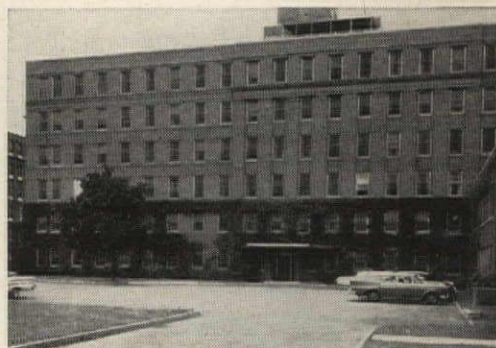
This hospital wing in Rochester, N. Y., was constructed in 1940.
