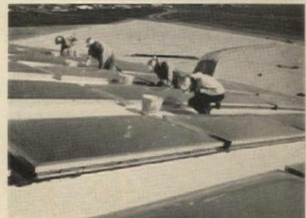
Top: Neoprene applied with pressure-fed rollers over glass roving. Above: Elastomeric tape seals joints. Below: Coating panels between skylights
