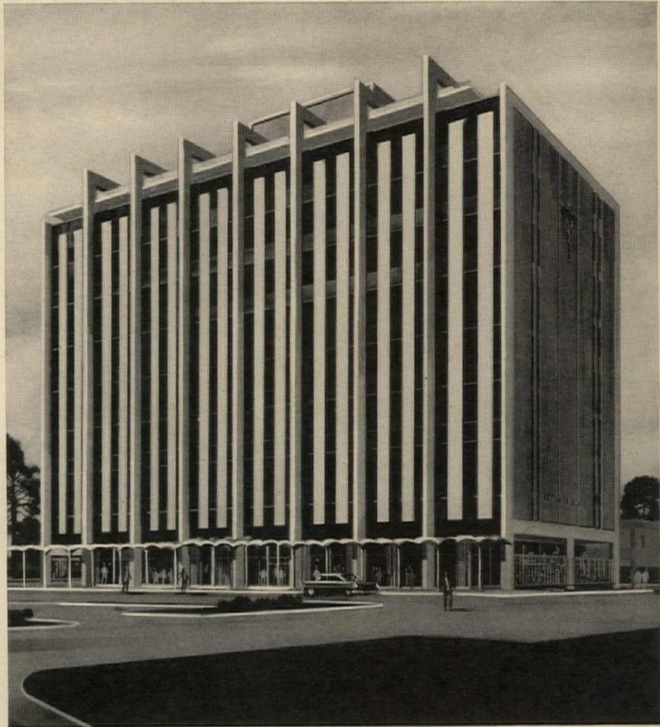
LOCKE MEDICAL BUILDING , Dallas, Texas. This modern medical center is cooled by a York centrifugal Turbopak water chilling system. Architect, Harold Berry; Engineer, Herman Blum Consulting Engineers; Mechanical Contractor, Natkin & Company.
