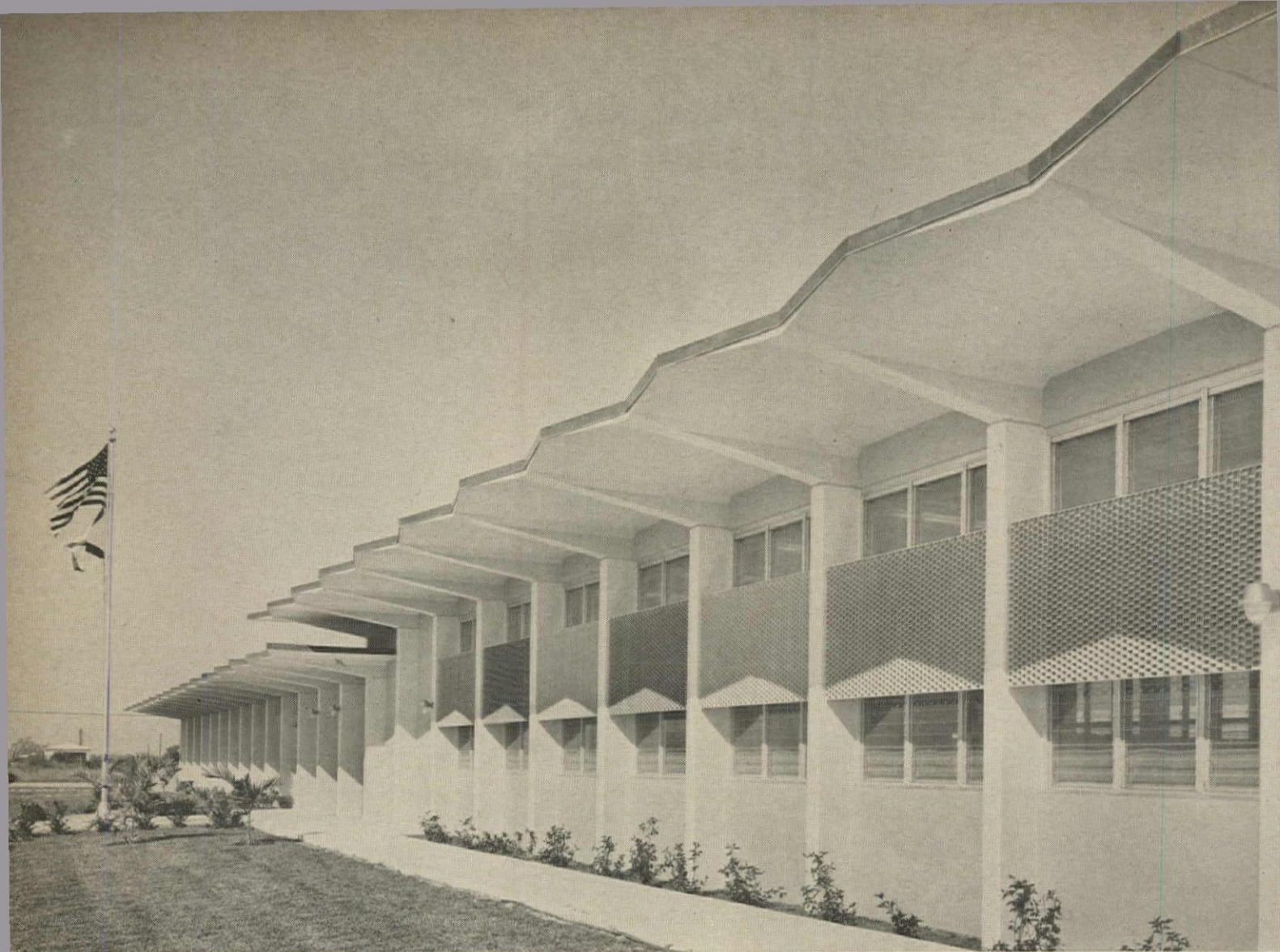
Architect: James E. Ferguson & Assoc., Coral Gables, Fla.
