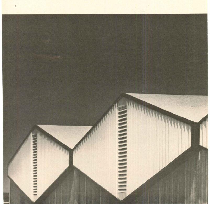
Despite its location on the shore of Lake Erie, exposed to extremes of weather, the siding on this new Transit Building will stay fresh and new-looking for many years. It's surfaced with a new and amazingly tough finish: TEDLAR\* PVF film.
