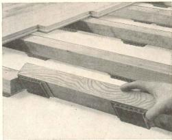
The PERMACUSHION Floor floats on special GR-S resilient cushioning pads attached to preservative-treated sleepers. These pads prevent contact with slab: no moisture transmission, unobstructed expansion control and complete air circulation beneath the flooring and sleepers. Power-nailing gives fast and proper installation.
