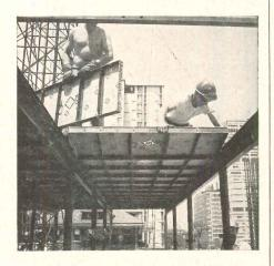
Symons Slab Shore System uses Symons standard Steel-Ply Forms, normally used for vertical wall forming, for all decking requirements. Material adaptability, ease of assembly, speed of erection and stripping are among its advantages over conventional flat slab forming.
