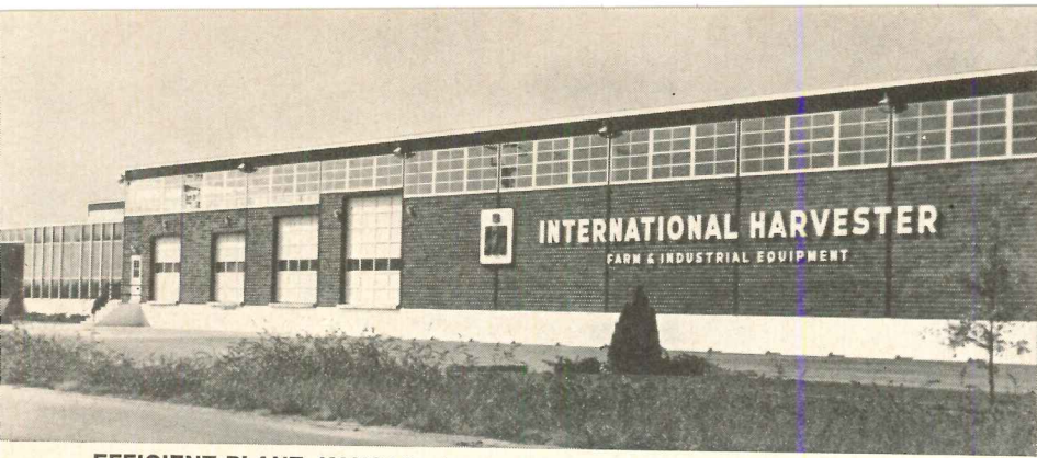
EFFICIENT PLANT, KANSAS —International Harvester, Wichita. Architect: Campbell Engineering Company. Prime Contractor: A. W. Soderberg Construction Company. Masonry Contractor: Kenneth D. King. Masonry Cement: United Cement Products Company. Concrete: Dolese Bros. Company.
