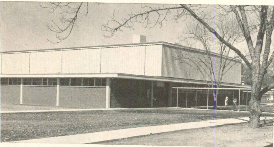
AIR-CONDITIONED SCHOOL, ALABAMA —Central High School, Phenix City. Architect: Ted Sztowitz, A.I.A. Prime Contractor: Williams Construction Company. Masonry Cement: The Raiford Coal Company.
