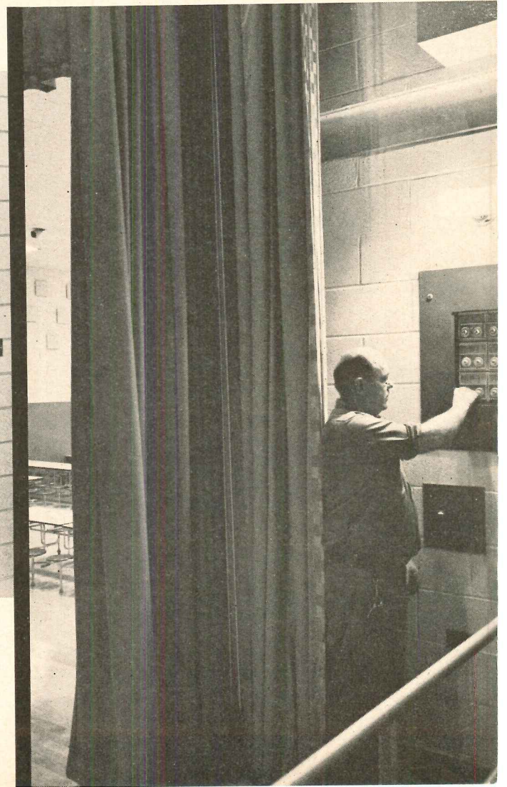
School's corridors and classrooms feature remote-control local light switches. Corridor switches are key-operated to prevent unauthorized persons from operating them.
