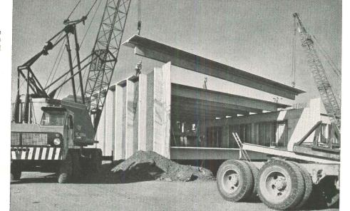
Fourteen prestressed single Tee beams form the roof; the same number are used for the floor. Roof Tees are 8' wide; range from 88.2' to 30' in length. Floor Tees are 73' long, 8' wide, 3' deep. The precast supporting columns are 34' high, 3' deep, 8" thick.
