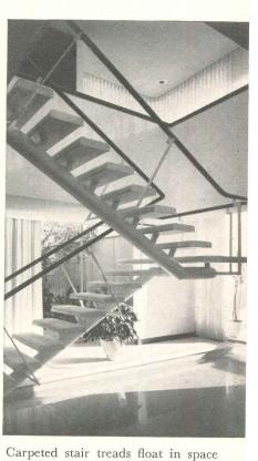
This spiral steel staircase connects three levels in a hillside home. It is composed of two strips of  $\frac{3}{8}$ -inch plate, 8 inches wide. Steps are 11-gage plate with edges bent upward to form a low box to hold a layer of concrete. Each step is supported by lengths of No. 4 reinforcing bar and welded to the two 8-inch strips. Handrails are 1-inch steel pipe. Architect-builder, Allyn E. Morris.
