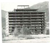
estimated at \$2.35 psf in concrete flat slab...it cost only \$1.94 psf using A36 steel and Bethlehem's Slabform steel centering over open-web steel joists.
