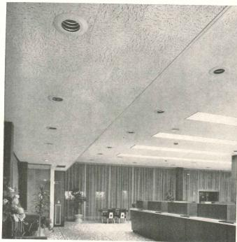
Fissured acoustical tiles for the ceiling in the Endicott Trust Building have a series of tiny holes for air supply
