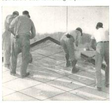
Lightweight "Incor" concrete roof slab is cast and finished over reinforcing.
