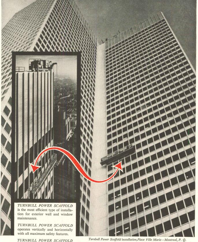
TURNBULL POWER SCAFFOLD is easily operated by safe push-button controls on roof carriage and workstage.
