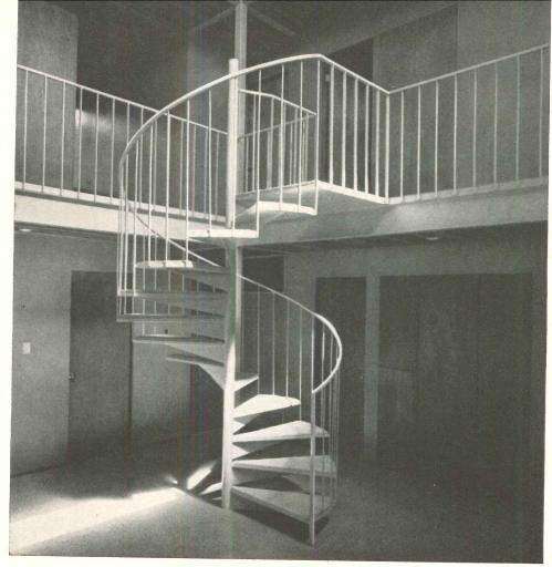
Two levels opening on a central court are connected with a spiral steel stairway in this home designed by architects Nelsen & Sabin. Treads, hanging from steel bars, are set into triangular frameworks of light steel angles.
