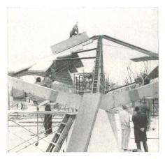
Insulating panels of polystyrene foam, which constitute the form for the thin-shell reinforced concrete roof, are fastened to high tensile steel wires.
