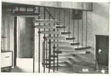
Architect J. Herbert Brownell designed this attractive stairway. Treads, composed of 3-inch thick laminated wood, are suspended on one end from  $\frac{3}{8}$ -inch diameter steel rods, and on the other end by 3-inch diameter pipe columns. The upper ends of the rods are welded to the bottom of one of a pair of 10 WF 15 beams which support the balcony.
