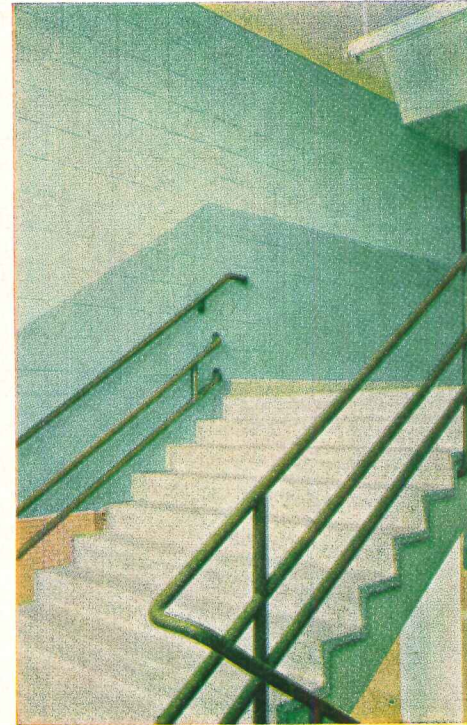
Stairwell is protected from heavy traffic by Glid-Tile.
