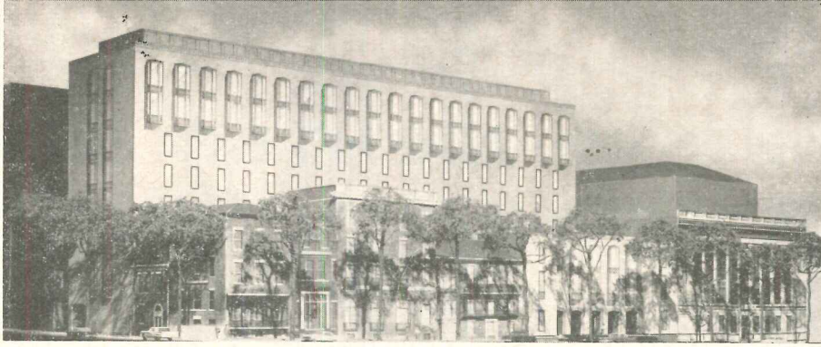
New Courts Building rises behind row of houses along Madison Place
