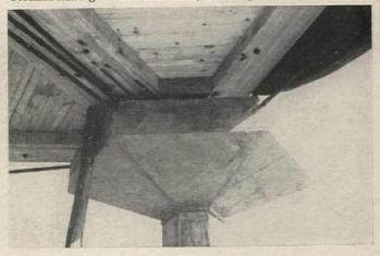
dependent, and is supported on the concrete columns by means of a knuckle joint connection which allows free rotation in all directions.
