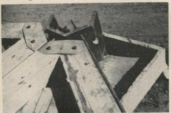
Column head gathers rainwater; discharges it into drain pipe
