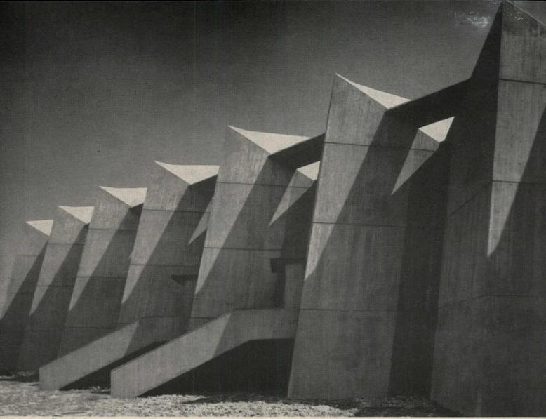
Tensile beams connect all unit arches together, pulling them toward the rear of the building
