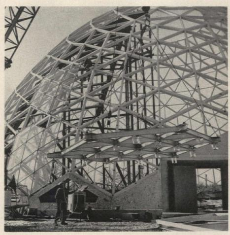
Lifting rig has just placed segment of aluminum and glass glazing on the precast dome. There are five basic glazing elements—three hexagons and two diamonds
