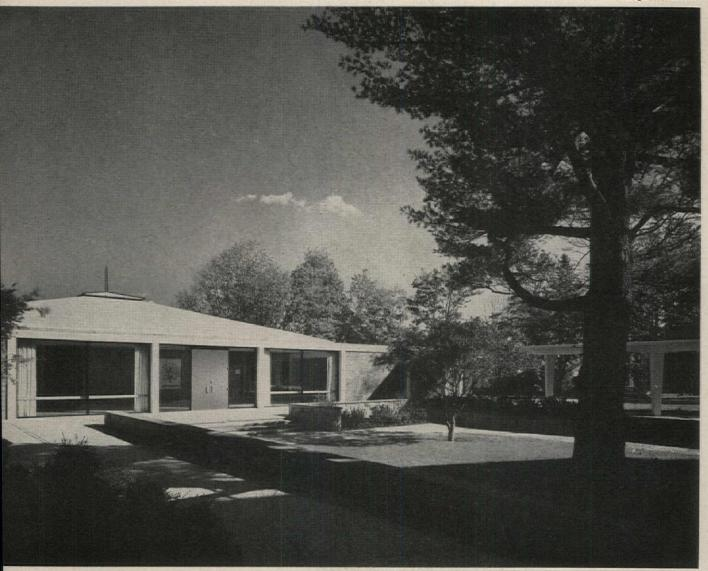
Parish hall has a pyramidal roof of reinforced concrete with central skylight. The structure is 72-ft square and seats 400
