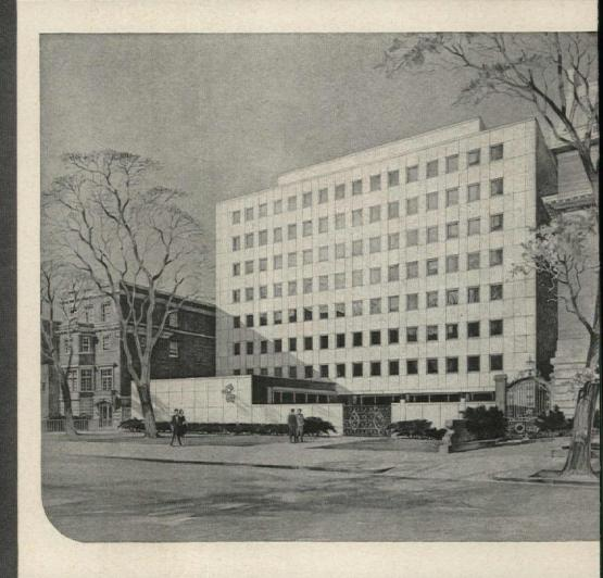
The Amelco Window offers many advantages . . . dual glazing with venetian blind between the panes of glass reduces solar heat gain by 65%. Just think of the savings in air conditioning equipment costs . . . and operating costs. Two inch air space and true thermal break in vent and frame offer 55% less heat loss in winter.
