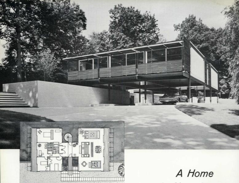
Two entry courts (small bridge crossing retaining wall, and circular stairway from carport), along with enclosed entry hall, divide the plan into two distinct parts-living areas to the east, bedrooms to the west.
