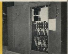
NEMA Size 6 starters, built by Square D's ECAM Division, control the motors and pumps which circulate chilled water through the air-conditioning system.
