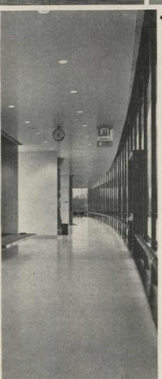
The floor tile in corridors and offices is Ruberoid/Matico Vinyl Asbestos. Over 300,000 sq. feet were installed.
