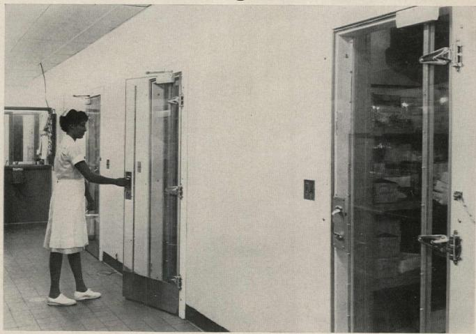
TRANSPARENT Jamison See-Thru acrylic cold storage doors installed in large kitchens of Marriott Motor Hotel provide easy access to cooler rooms.
