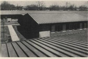
num with a uniformly deposited coating thickness of approximately .002 in. per side—twice the thickness of a commercial hot dipped zinc-coated steel. General surface corrosion resistance of the coating in normal atmospheric exposure is similar to 1.100 aluminum.
