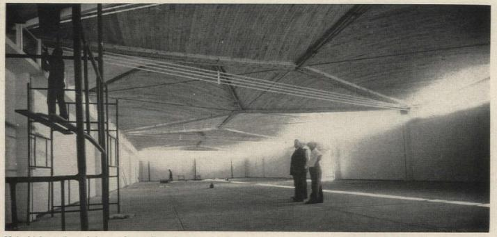
Main, high-tensile steel ties run diagonally and peripherally between columns to take thrust of the triangular roof panels
