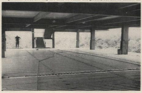
on each side. Shear studs were attached to the girders—with the exception of cantilever ends—and to most of the beams. Formed steel decking was used as a permanent form for the concrete floor.
