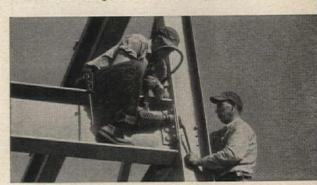
SAVE CONSTRUCTION TIME with Republic's New Heavy Head High Strength Bolt Assemblies. Two-man team replaces costly erection crews. When wrenched up tight, Republic High Strength Bolts provide a vise-like clamping force which transfers loads by friction to the structural members. Fatigue life is improved. Joints are stronger than connections where loads are carried in shear. Send coupon for illustrated folder.
