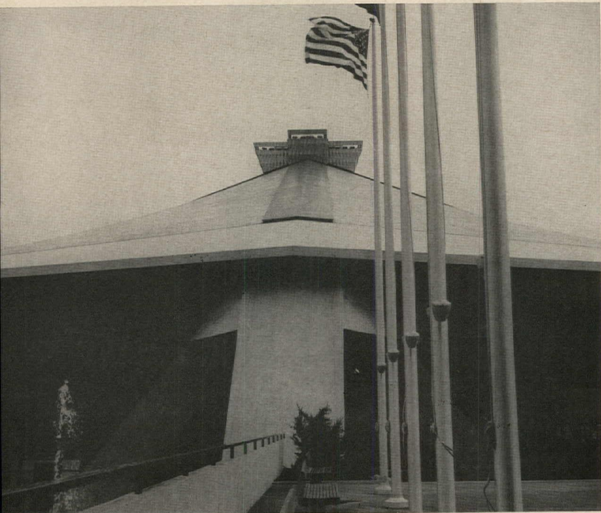
Strong structure, simple form of Paul Thiry's Coliseum for State of Washington, seen close-up from walk on top of wall behind Everett DuPen's fountain
