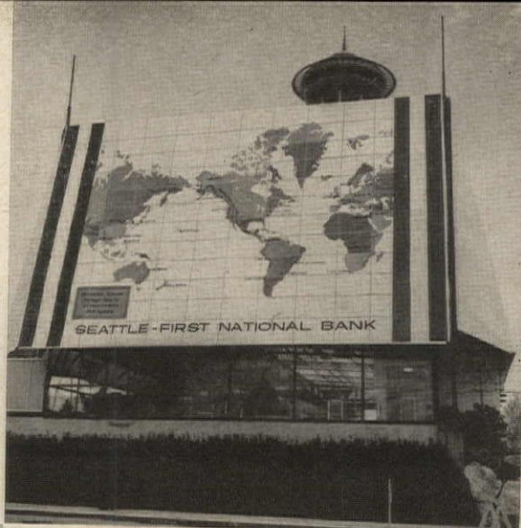
Canvas over a steel frame—height and prominence without expensive structure. Seattle First National Bank; Paul Thiry, architect
