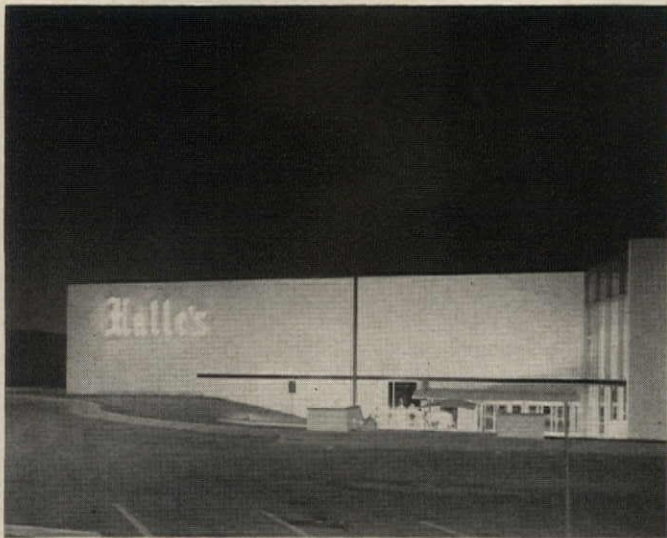
White store facade is floodlighted with two 1000-watt incandescent units concealed from normal view. Luminous tube sign in blue identifies store while dark stripes frame the entrance
