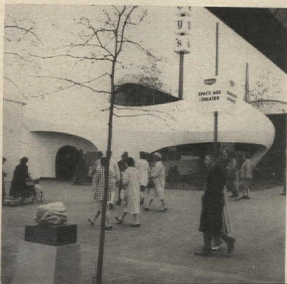
Plastic form shell for Nalley's pavilion, concrete pneumatically applied on frame of reinforcing rods and metal lath. Paul Thiry, architect
