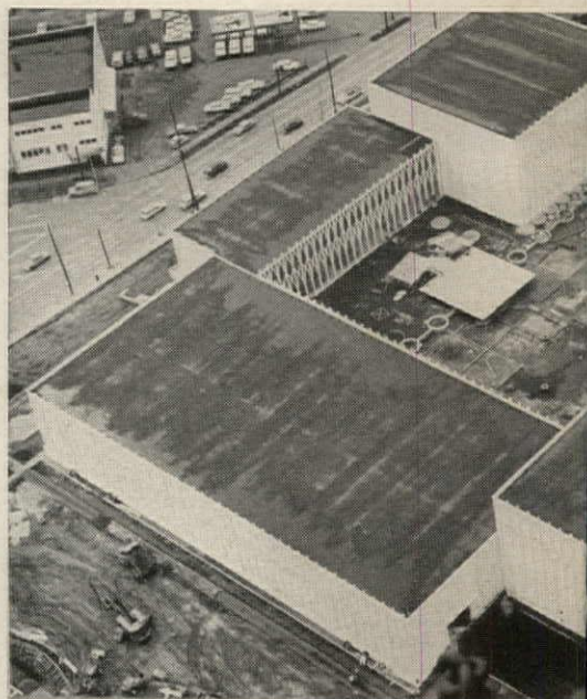
U. S. Science Pavillion. The six buildings and five 100' arches are of prestressed concrete from the ground up. This new concept in construction offers freedom for aesthetic expression.
