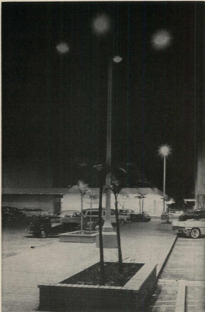
Concrete poles with water-polished finish carry out motif of masonry planters, support one to four streetlight luminaires. Note the bumper-high pole bases
