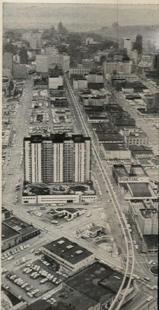
Monorail Transport System. Rubber-tired 4-Car trains will carry 450 passengers on prestressed, hollow concrete track cast in 120 feet lengths. Speed 97 seconds per trip. Said to be the solution to mass transportation in the future.
