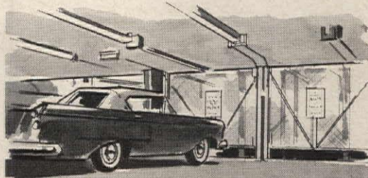
Automatically-operated, upward-acting, expanded-metal gates by "OVERHEAD DOOR" are used in this pigeon-hole parking structure at Columbus, Ohio. Representing the newest in car-park automation, this driverless "file system" depends on The "OVERHEAD DOOR" for swift, automatic handling.
