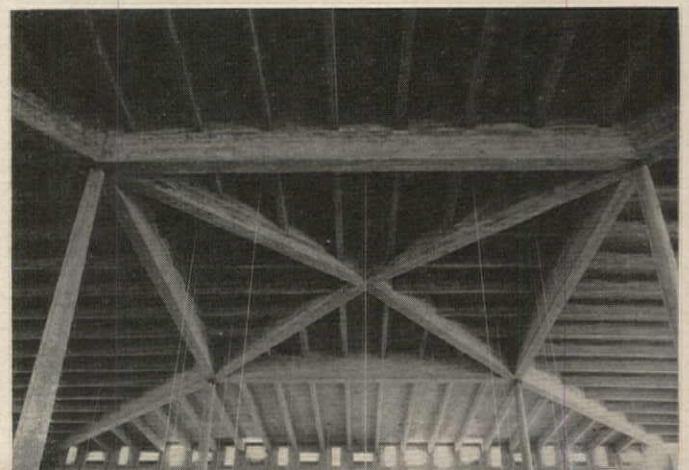
Ceiling above sanctuary
