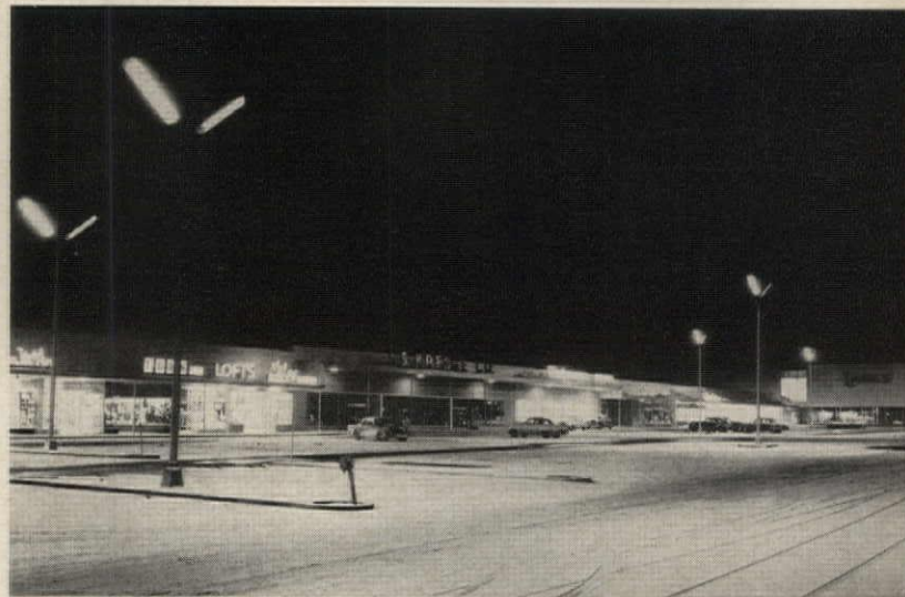
Fluorescent luminaires designed for area lighting, although somewhat more costly than mercury units, do provide opportunity for a change of pace or color in parking areas
