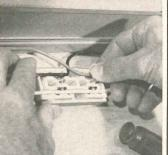
"Outlets can be installed wherever wanted, without cutting or stripping wires. Insulation-piercing terminals do a good job.
