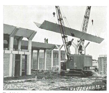
The folded plates for the cafeteria roof are 5'3'' wide,  $2\frac{1}{2}''$  thick. Along the length of the building they make three spans of 60, 48 and 60 feet, with an 8' overhang at each end.
