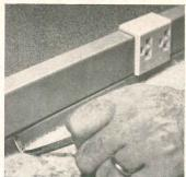
"Changes, additions or replacements are easy with G-E FLEXWAY Wiring. Wires can be exposed in seconds; covers snapped back on.
