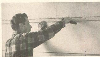
KEYSTRIP can be used as a reinforcement for plaster in a space too narrow for strips of gypsum lath. A full bond of Keystrip to the plaster is assured. Keystrip also adds strength to points of stress above doors and windows.
