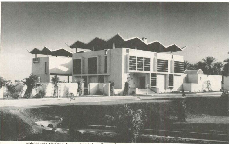
Ambassador's residence. It is protected from the sun by a hyperbolic paraboloidal parasol, which forms a reflecting sun shade and allows free air circulation below. Servants wing to right of photograph
