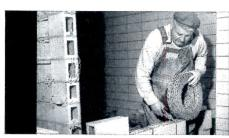
Fine tile work demands uniform mortar joints. Only Keywall can be lapped without lumping in mortar joints. That's why W. E. Broady & Sona found Keywall the neatest solution for reinforcing all tile work in the new Indianapolis City-County Building.
