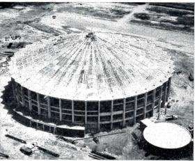
Precast concrete sections, poured at the job site on Tectum Form Plank forms, are lifted by crane to the roof level. Building: Coliseum for State of Mississippi, Jackson; Architect: Jones & Haas, Jackson.
