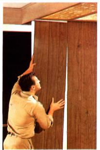
For fast installation, Marlite Random Planks ( $\frac{1}{4}$ " x 16" x 8') are tongued and grooved-assure a better finished job.
