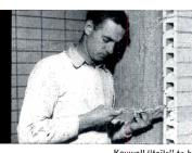
Keywall "tails" to be tiedin later. You can appreciate this advantage when continuous reinforcement is needed, even though some wall sections must be left unfinished for other work. Only Keywall is flexible enough to accommodate variations in mortar joint levels.
