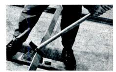
Switches and outlets can be located wherever needed, in General Electric Flexway Wiring. Devices fit onto a base channel, and the spaces between them are closed with raceway covers, easily cut to length with a special tool.
