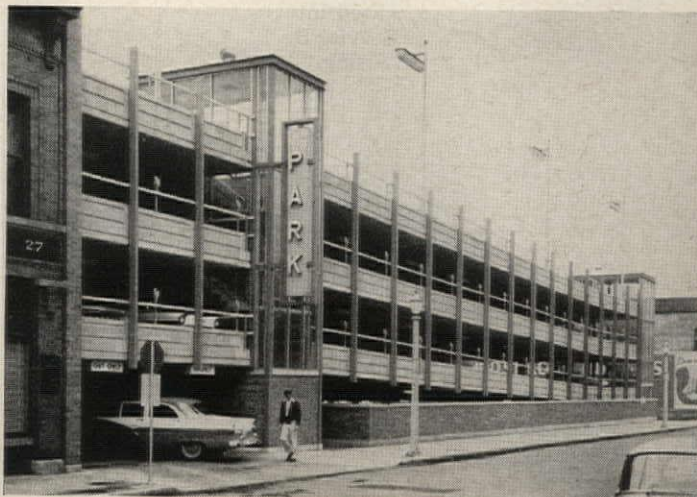
Parking structure in Oshkosh, Wis. , is the first of its kind in the Midwest to be built with lift-slab construction. Owner: City of Oshkosh. General contractor: William Warner Construction Co., Oshkosh. Architectural and engineering work: A joint venture by Sandstedt-Knoop-Yarbro, architects, Oshkosh—and Charles Nagel and Associates, Inc. architects and engineers, Milwaukee. Lifting Contractor: Great Lakes Lift-Slab, Chicago.
