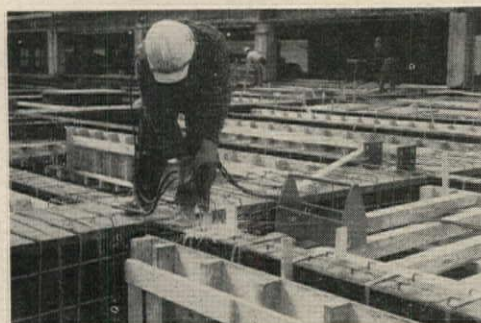
Above: Hundreds of 2¼-in. high shear connectors have been welded to steel framing on an upper mechanical floor. Full advantage can be taken of composite action because concrete floor slabs are used at mechanical levels. Below, right: "L" type shear connectors are welded to top flanges of steel; note closeup
