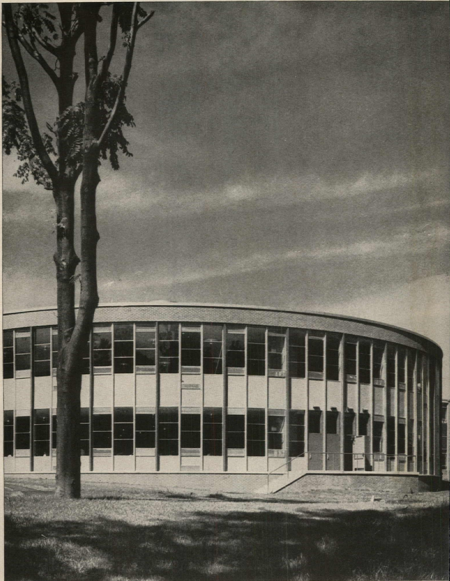
Great Neck Junior-Senior High School, North Hempstead, L. I., New York. Architect: LaPierre, Litchfield & Partners (Alfred Hopkins & Assoc.). Contractor: Peatty & Fuhrman, Inc., New York, N. Y. Photograph by: C. V. D. Hubbard.
