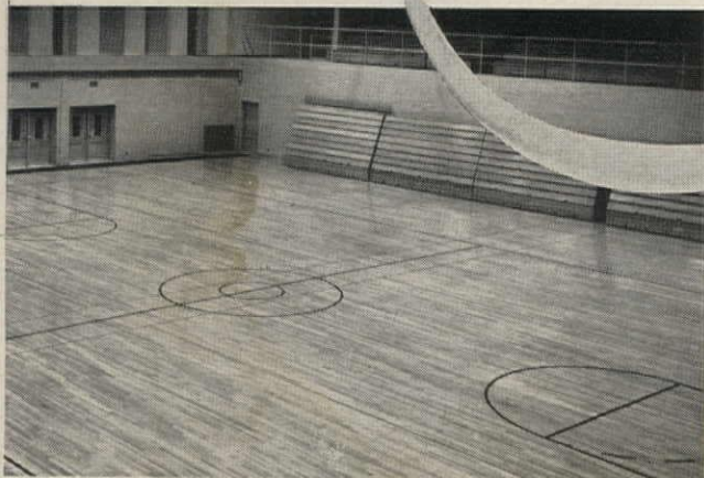
This "Air Thrust" Pneumatic Hard Maple Floor System was installed by Chas. H. Anderson Floors, Inc., Chicago, Ill., in the Prospect Heights Field House, Arlington, Ill. It is an example of a fine hardwood floor system . . . well made . . . well laid.
