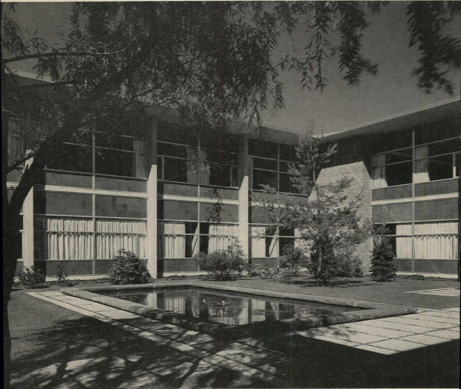
One of two courtyards. Spandrels are panels of insulated gray slate. Face brick is a warm pink. The multi-colored aggregate exposed as a result of the bush hammering was carefully selected for color and size from local sources
