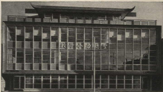
St. Theresa Chinese Catholic Mission, Chicago, Illinois. Architect: Kefer and Cronin, Chicago, Illinois. Contractor: Ashland Construction Co., Chicago, Illinois. Photograph by: Hedrich-Blessing.
