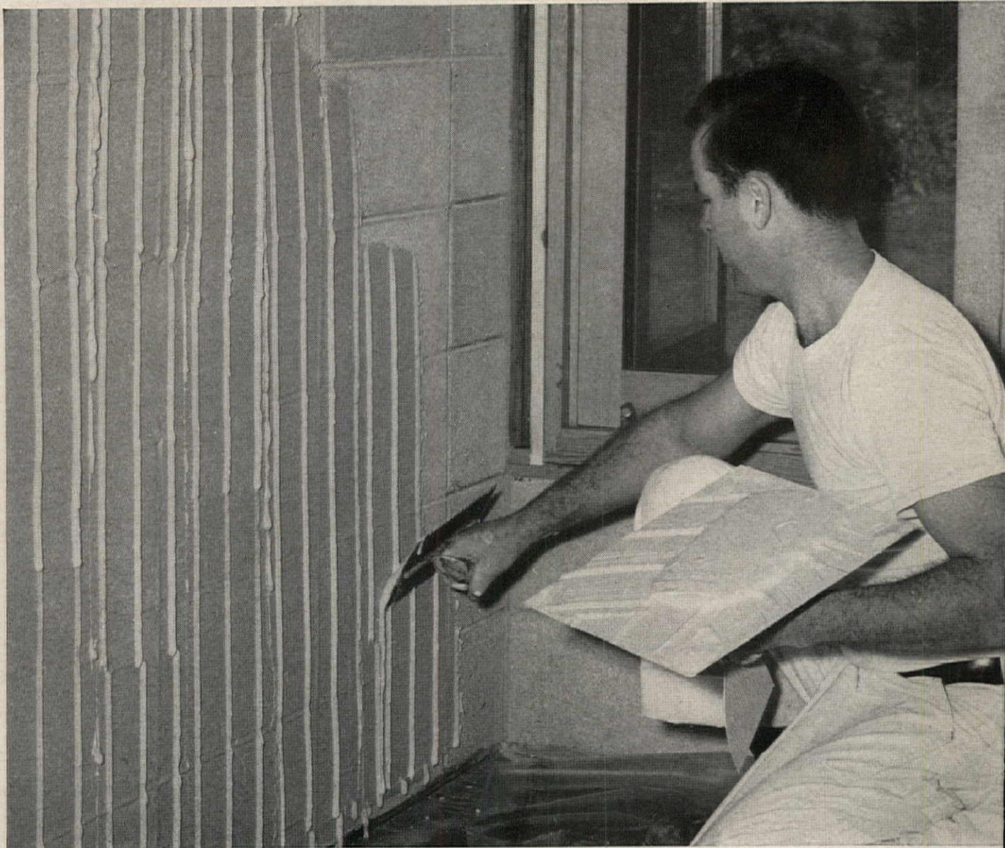
After Styrotac™ bonding cement is applied to either the wall or to Styrofoam, the insulation is pressed in place (center). After overnight setting, gypsum wallboard is either spot-coated or notch-trowelled with Styrotac and pressed in place over the Styrofoam insulation (right).
