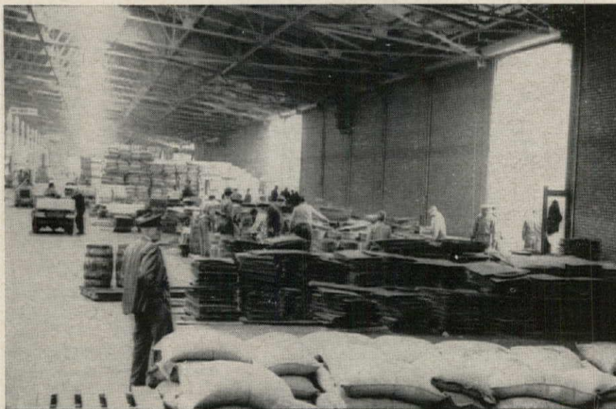
Moore-McCormack Lines Inc. Brooklyn Terminal, New York Arch./Engr. — Miles A. Gordon Contr. — Nadel-Baxendale, Inc.
