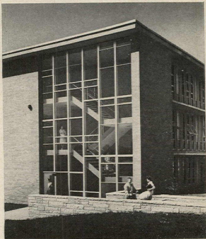
Interesting design pattern is achieved with a combination of Pittsburgh Polished Plate Glass.
