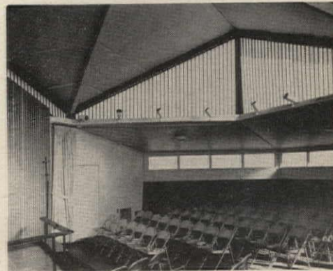
Built-in pew at back conceals ductwork
