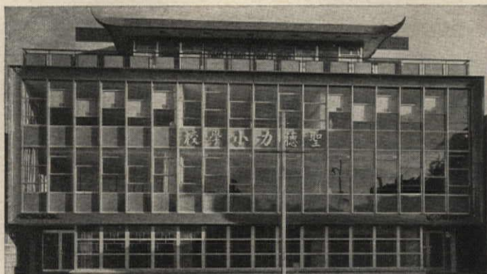
St. Theresa Chinese Catholic Mission, Chicago, Illinois. Architect: Kefer and Cronin, Chicago, Illinois. Contractor: Ashland Construction Co., Chicago, Illinois. Photograph by: Hedrich-Blessing.
