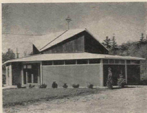
Exterior as it looks when completed
