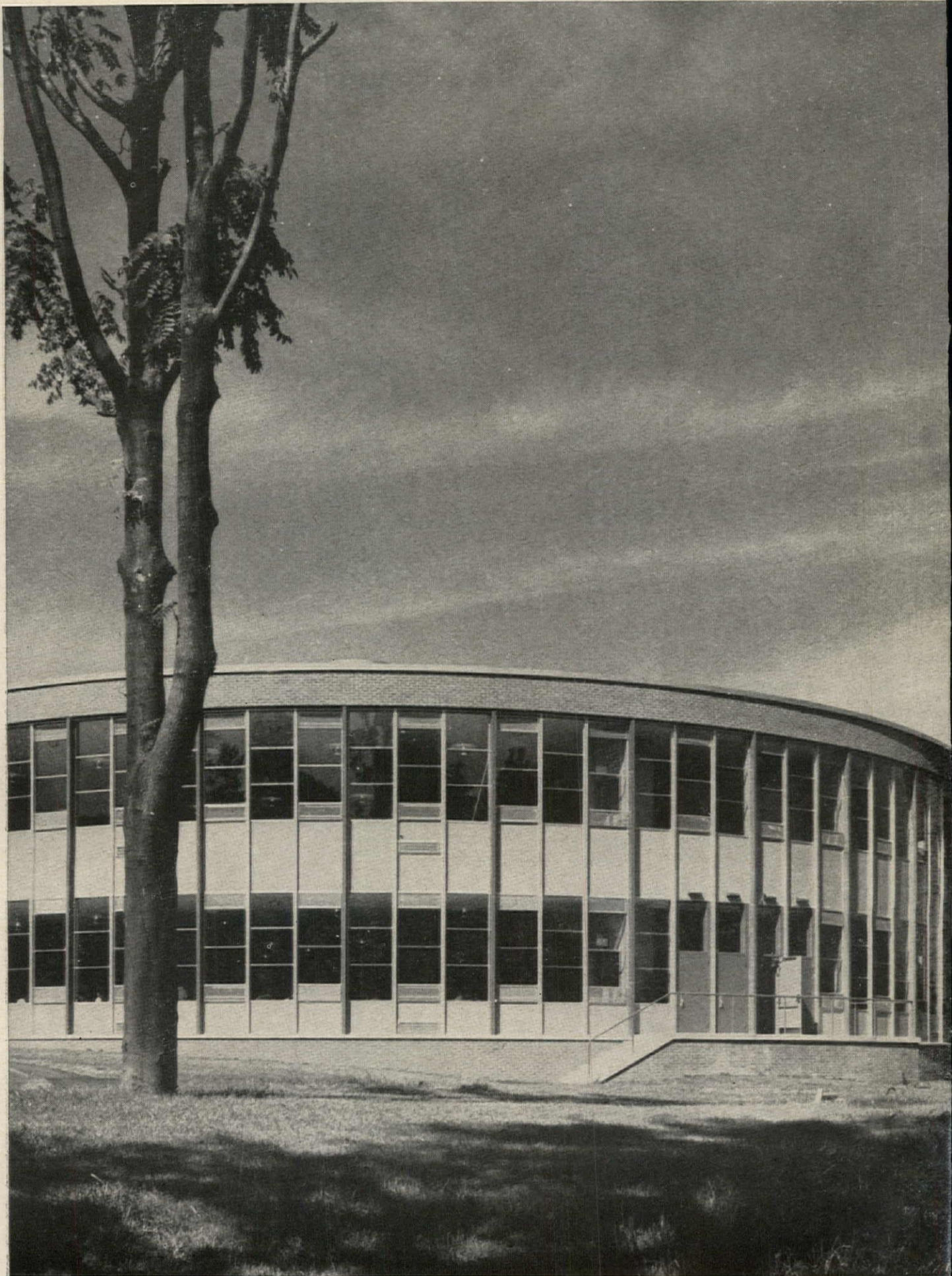
Great Neck Junior-Senior High School, North Hempstead, L. I., New York. Architect: LaPierre, Litchfield & Partners (Alfred Hopkins & Assoc.). Contractor: Pealty & Fuhrman, Inc., New York, N. Y. Photograph by: C. V. D. Hubbard
