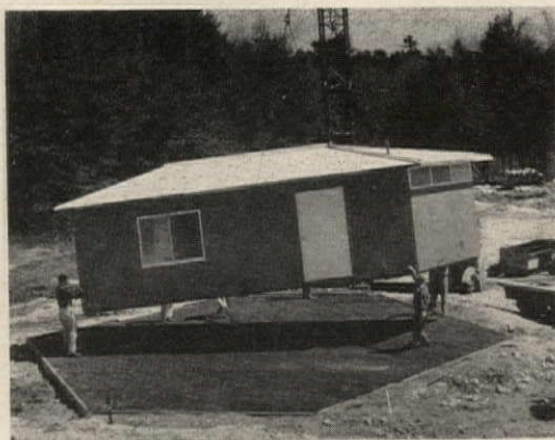
Kitchen, utility unit is factory assembled
