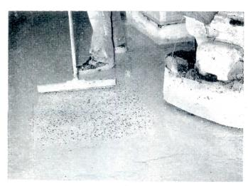
Conventional grinding equipment is used to smooth the trowelled surface. This is usually begun the next day after the pour when the floor has had sufficient time to cure
