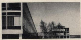
Over 82,000 sq. ft. of FOAMGLAS insulates these glass spandrel panels at the Connecticut General Life Insurance Building, Bloomington, Conn. Fabricated right on the job, FOAMGLAS protects the steel from air and moisture damage while it serves as the backing for the metal flashing that rings the building.
