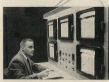
One "Electrionic" recorder provides a permanent 24-hour record of temperatures at as many as 24 different points in the building.
