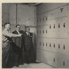
A. J. Eversmann, Maintenance Superintendent of WAVE, inspects the modern and compact Westinghouse building-type switchboard with R. A. Schlaug and M. D. Bornstein, both of Bornstein Electric Company. Westinghouse AB De-ion® circuit breakers distribute and protect all power circuits in the studio. Provision is made to install additional breakers when required in the future.
