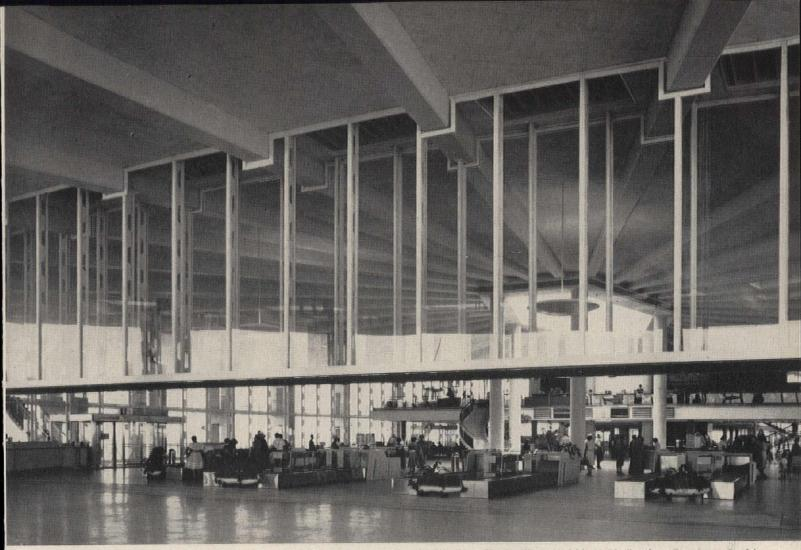
89-ft wide, 7-ft deep air entrance for Pan American passenger terminal in New York; Tippett-Abbett-McCarthey-Stratton, Architects & Engineers. Air reaches supply grille through a 23-ft high glass-enclosed plenum to make the full opening transparent.
