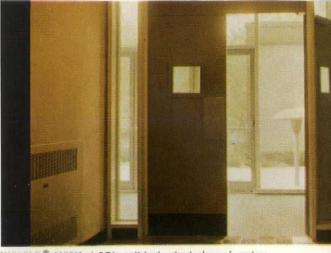
NUWELD® MESH. A-SG's polished, wired glass of modern design is extensively used in the GEICO building. It was specified because of its fire-retarding properties—for enclosures around computer installations and other valuable equipment, and for corridor partitions. Its unobtrusive linear pattern complements the distinctive interior decor.
