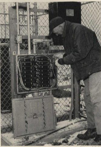
New THW wire insulated with Geon is used in sizes up to 3/0 AW G at this new Sohio plant. Wire is made by the Paranite Wire and Cable Division of the Essex Wire Corporation, Marion, Indiana. B.F.Goodrich Chemical Company supplies the Geon vinyl,
