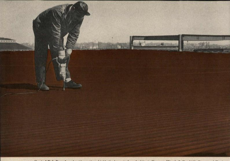
Coated Fab-Form's red oxide coating shields the base steel from corrosive elements in concrete. Here, on the roof of Looman Associates Office Building in Trenton, N. J., coated Fab-Form was installed by a four-man crew in just one day.
