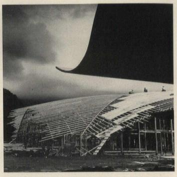
Conventional formwork was built for the shell and, while not an engineering requirement, the contractor elected to pour it in one piece. In the first few weeks after removal of the forms the center deflected approximately 2 in. The discontinuous edge deflected about 3 in. downward at the center of its span, and rose 1 in. at the quarter point
