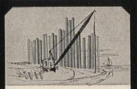
INLAND BEARING PILES AND STEEL SHEET PILING are used in foundations, retaining walls, coffer dams and other excavating and supporting jobs.
