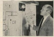
A single "Electrionic" eye-level indicator can be used to check temperatures at an unlimited number of points throughout a building.
