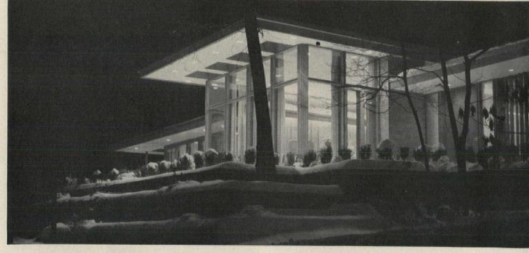
GREENE RESIDENCE, Short Hills, N. J. All exterior window walls were constructed of prefabricated modular load-bearing
