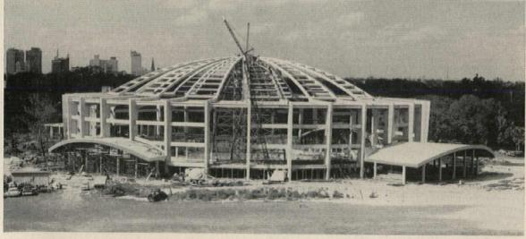
Clear span at base of structure is 302'. Height to center roof ring is 95'. Height to perimeter roof is 65'. Circular roof rib radius is 250'. Two of three entrances take shape in foreground.
