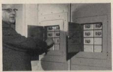
G-E master selector switches at ends and center of each floor control lighting separately for each ½ floor. Building contains 2000 fluorescent lamps.
