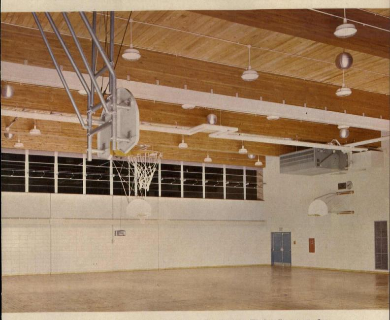
In natural finish, Glulam beams and Tim-Deck by Timber Structures, Inc.
