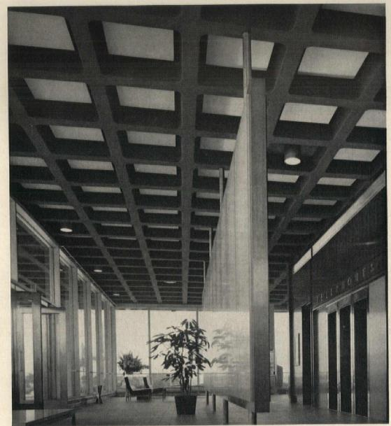
The main corridor of a Fred Harvey Oasis Restaurant on Tri-State tollway near Chicago, illustrating a dramatic ceiling treatment possible with Steeldome construction. The exposed concrete waffle ribs are painted charcoal gray, sounding a new note in decor motif.
