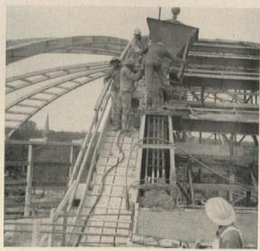
Placing concrete for roof ribs high above coliseum floor.
