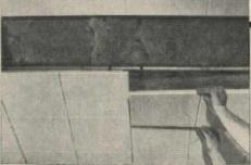
Aluminum panels of Burgess-Manning Heating, Cooling and Acoustical Ceiling, re moved to show hot water coil and acoustic blanket.
