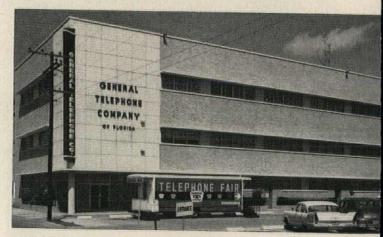
TELEPHONE EXCHANGE—General Telephone Company of Florida (Sarasota) uses Cat Electric Sets for standby power. Exchange has 30,000 dial telephones. Long distance facilities are provided by a 48-position toll board. Out-of-town connections are made through 120 microwave circuits as well as underground cables.
