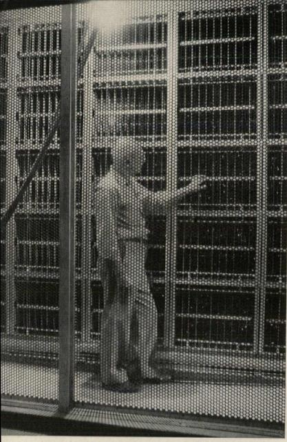
Jacob Dietrich views Westinghouse PRECIPITRON®, the Electronic Air Cleaner which removes up to 95% of all dirt particles, smoke and pollen in the air circulating throughout the building. This improves working conditions and also protects employe's health. The PRECIPITRON traps microscopic particles that cause streaks, smudges, damage to interior furnishings and office equipment, thereby reducing cleaning and maintenance costs.
