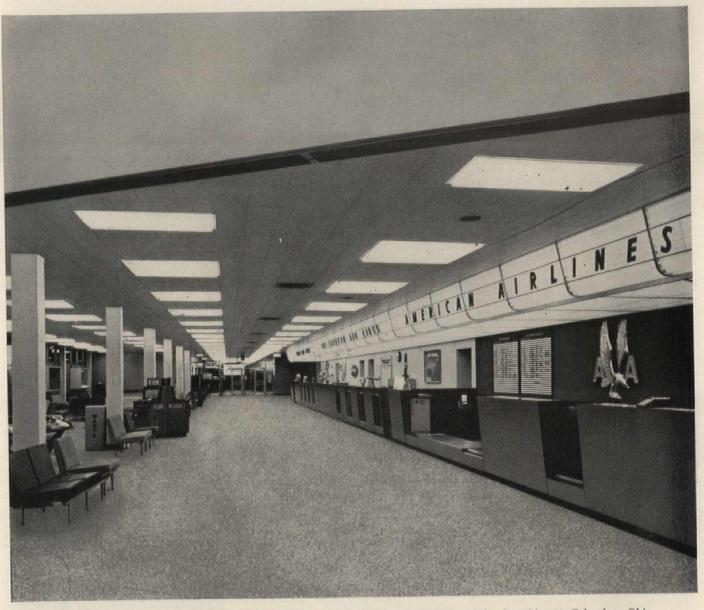
Ceiling diffusers, counter lighting and identification panels of PLEXIGLAS at Port Columbus Airport, Columbus, Ohio
