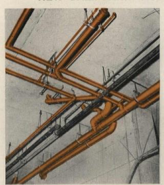
CLOSE WORK LIKE THIS is possible only with copper tube. Water and drainage lines hug the ceiling, giving ample basement headroom. Even in tight quarters, connections are easy to make. Sizes in this photo range from ¾" water lines to 4" for drain and vent lines.
