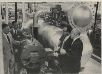
One of two Westinghouse 200-hp Life-Line motors which drive compressors in air conditioning system, Westinghouse motors from 1 to 200 hp were specified for all auxiliary equipment drives. Having a single source of supply simplifies maintenance and spare parts problems for operating equipment. Discussing the installation are J. P. Anderson; C. E. Pickering; J. O. Unthank; and Harold Stebbins, Vice President, Bankers Life of Nebraska.
