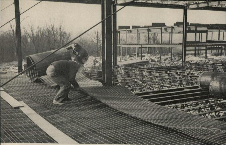
Quickly, easily Steeltex goes down at superbly designed Canevin High School, Pittsburgh, where 60,000 square feet of Steeltex support concrete floor slabs, Architect: Celli-
