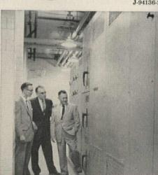
C. E. Pickering, J. O. Unthank and J. P. Anderson are shown in front of Westinghouse 1500-kva dry-type ASL power center. This power center steps incoming voltage down from 5 ky to 277y/480 for distribution through three Type DB-50 air circuit breakers.
