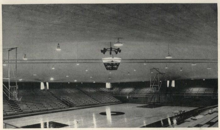
The "tent-like" dome of this hyperbolic paraboloid design utilizes acoustical values of Tectum form plank to absorb sound\*.
