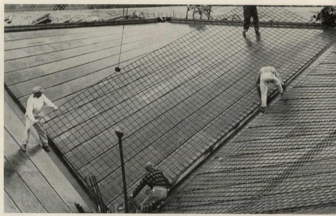
A 700-pound USS American Welded Wire Fabric Mat is placed on one of the six umbrellas. It is Style 6 x 6–5/0 and 5/0. The mats are lapped and
