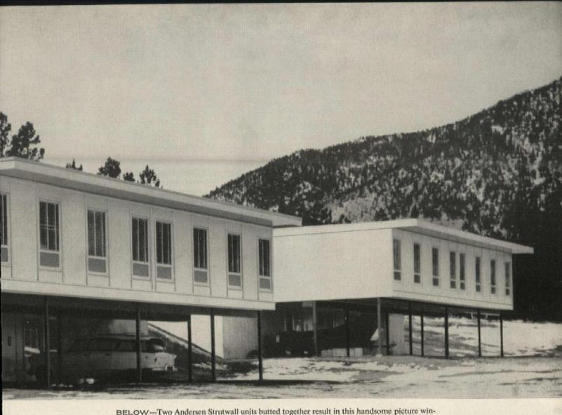
BELOW—Two Andersen Strutwall units butted together result in this handsome picture window effect. Lower operating sash are awning type, Permit ventilation even during rain storms.
