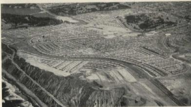
Figure 4. Contrasts present smoothly graded residential area with original rough site. Some houses are founded on fills up to 80 ft thick
