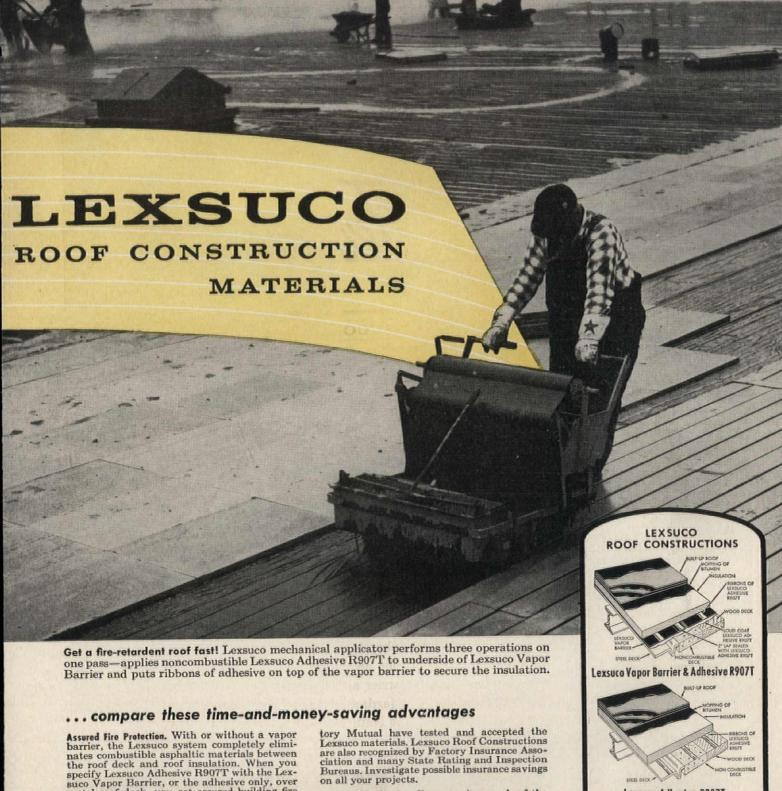
Assured Fire Protection. With or without a vapor barrier, the Lexsuco system completely eliminates combustible asphaltic materials between the roof deck and roof insulation. When you specify Lexsuco Adhesive R907T with the Lexsuco Vapor Barrier, or the adhesive only, over metal roof deck, you get assured building fire systems.
