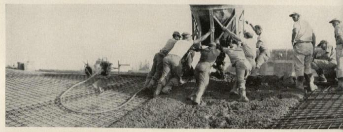
Concrete is poured from the top, worked down toward the center, vibrated and rough screeded. A 3" topping of perlite insulating concrete was poured directly on the rough surface. Less concrete is needed for any
