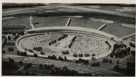
The new passenger terminal building at New York's LaGuardia Airport is being constructed in phases, with completion scheduled for 1962. The 1250-ft-long structure, about 100 ft deep, will provide some
