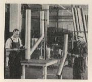
IN THE SHOP, the Contractor for the Kaiser job prefabricated 354 sub-assembly styles using copper tube by Chase.
