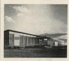
The building was, naturally, designed to exhibit as many uses of ceramic tile as possible. Both the mortar and mastic techniques were used in installation. Tile panels ranging from 15 to 200 sq ft cover the exterior of the steel-framed structure. The panels, in blue, red, yellow, and tan, are large outside laboratory areas and smaller near the office-area windows. Mosaics are used on the undersides of the three entrance canopies. The porches and walks are also tiled.
