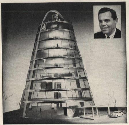
**NO COLUMNS!** In an unorthodox application of stress principles to multi-story construction, Architect Seymour Rutkin of New York has eliminated encumbering columns, achieved maximum space flexibility.
