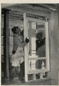
Andersen Strutwalls afford tightest possible joining of windows and walls. Insure all-weather comfort. Cut installation time as much as ½ over conventional windows.
