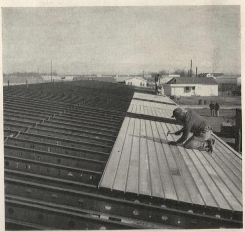
STEELDEK was nailed to the Penmetal steel joists. Light weight makes it easy to handle. The rigid sheets fit quickly into place.
