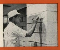
PELASPAN 8 Insulates curtain walls. New expandable polystyrene beads provide excellent insulation for curtain wall panels. When expanded, Pelaspan 8 conforms to any shape, forms durable barrier to heat and moisture.
