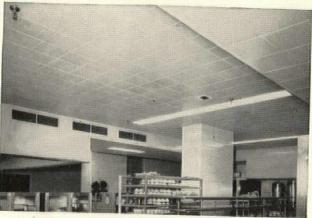
Service area, in new section of hospital, with Grinnell Pendent Sprinklers in view.
