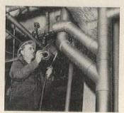
ON THE JOB, installation of these sub-assemblies is quick and easy, using solder joints that are leakproof and pressure-tight.
