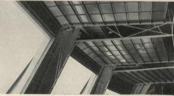
Doors in upward position at shop entrances. Doors used in this installation are fully automatic. However, The "OVERHEAD DOOR" is available to architects custom designed for any requirement; variety of materials, weights.
