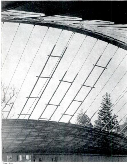
Left: cables are standard bridge strand. Roof deck is constructed of random lengths of 2- by 8-in. tongue and groove treated wood planks nailed to a pair of 2- by 6-in. nailing strips which in turn are bolted to the cables
