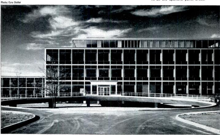
Spandrels are faced with gun metal gray Spandrelite\* backed by a 1" air space and  $1\frac{1}{2}$ " FOAMGLAS insulation. The insulation's unusual strength and rigidity permitted its use without special extra supports. Blocks of cellular glass insulation were also used to fill in the web between the flanges of the steel structural members of the new Connecticut General Headquarters. \*Manufactured by Pittsburgh Plate Glass Company
