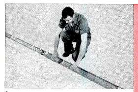
Assemble the Uni-Race • The exclusive Gibson Raceway, known as the Uni-Race, can be assembled on the floor in lengths up to 200 feet. The four or eight-foot sections are joined by telescoping couplers which provide a smooth, rigid union of the sections and are fastened with self-tapping screws.
