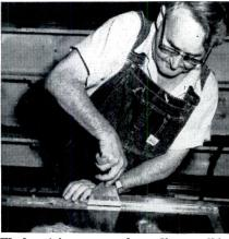
Worker trims excess from fiber caulking packed between "sandwich" and frame
