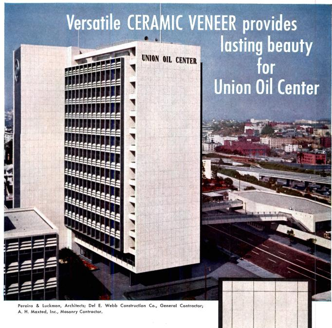
The new Union Oil Center in Los Angeles is distinguished by the effective use of light-grey adhesion type Ceramic Veneer.
