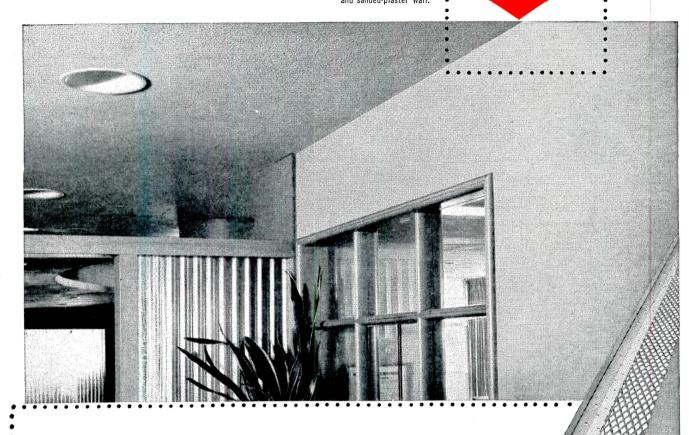
Milcor Casing Bead separates acoustical and sanded plasters
