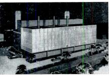
Boiler House addition, Provincial Hospital, Essondale, B. C.; Toby and Russell, consulting architects; Swanson Wright and Co. Engineers Ltd., engineers; Beaver Construction Ltd., Vancouver, general contractor. Addition is reinforced concrete to main floor level; above, steel structure with aluminum and glass curtain wall
