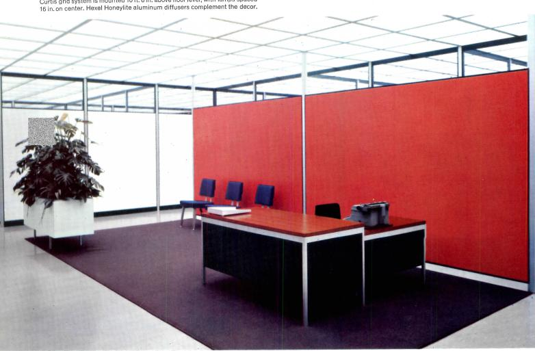
Vast expanse of office areas can be altered to any size or shape without destroying ceiling pattern or lowering lighting standards. In this special Curtis grid installation, aluminum materials were used throughout. Maintenance advantages are: ease of relamping, ready access to wiring, and simple replacement of the ballasts.
