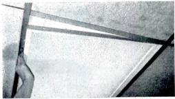
Easy access cuts maintenance time, costs Simple push upward releases hidden latch. Concealed hinging swings shielding down, holds it throughout cleaning and lamp changes. Each fixture is individually fused.
