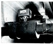
one in the return main. The total Btu's consumed are determined by the integrator, which mechanically multiplies the temperature difference by the weight of water used, and registers the cumulative result on the face of the meter.
