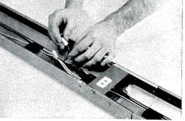
2 Wire the Uni-Race • Branch-circuit wires are laid in the Uni-Race and connection is made at each built-in receptacle. The receptacles will later receive the plug that is built into each fixture. The Uni-Race, U. L. approved as a raceway, has a capacity of five No. 8 AWG wires or eleven No. 14 wires.
