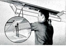
4 "Plug In" the Fixtures • The fixtures are merely "plugged in" on the Uni-Race. Hooks on the fixture engage in slots on one side of the Uni-Race, acting as hinges. The fixture is swung closed and latched. The built-in plug on the fixture automatically connects with the receptacle in the Uni-Race.
