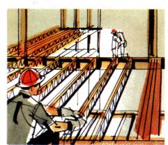
**Open-Web Joists**—Complete series of shortspan and longspan types, and accessories
