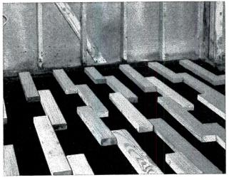
Lay screeds at right angles to proposed direction of flooring, 12" on centers with ends lapped 4". Staggered pattern helps to provide good nailing surface.
