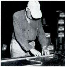
Pre-formed neoprene gasket is inserted in joint over caulking fiber insulation
