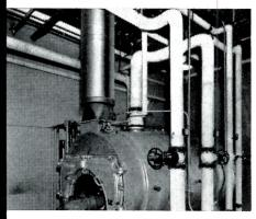
Installing this stack is quick and easy. Three-foot sections are simply cemented atop one another with acidproof cement.
