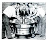
The foot-controlled sprayhead serves 8 to 10 but the total amount of water is no more than for a conventional wash basin.
