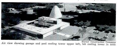
Air view showing garage and pool cooling oratory rooms. The reactor is a "stock" 5 megawatt pool type using 4.5 kg of Uranium and having walls up to 10 ft thick at the hot end. Air conditioning maintains a slight neg-
