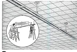
Hang the Uni-Race • The rigid Uni-Race is easily lifted and hung in any of several diferent ways. Lengths up to 200' can be hung as a unit if supported every 24' while being raised to mounting position. When the branch-circuit connection is made, the Uni-Race is ready for the fixtures.
