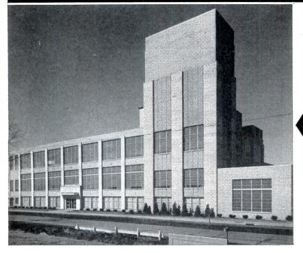
New factory of American Chicle Company, Rockford, III. where 14,000 sq. ft. of Coolite Wire glass, Glare Reduced, combines heat absorption with protection.
