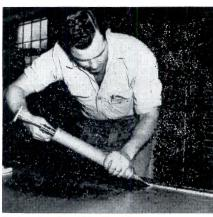
Strip of polysulfide liquid polymer, gunned on over fiber and gasket, completes seal
