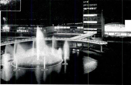
• "Gateway to the Stars"—at Idlewild Airport—is a curving reinforced concrete promenade which connects with a prestressed concrete bridge leading to the Arrival Building.
