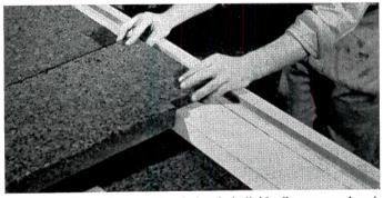
**Insulation**—Each block of insulation is individually measured and cut to give maximum insulation efficiency.
