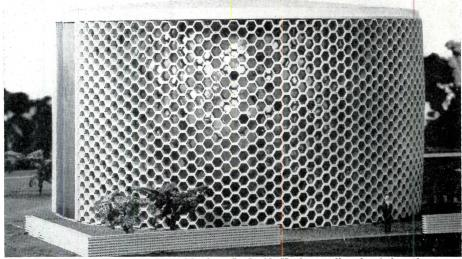
Chapel for Temple Emanuel, East Meadow, L. I., N. Y., has walls of reinforced precast concrete half-hexagonal units, to be laid up in a running bond. This continuous structural skeleton will be filled with colored glasses. Roof structure is still under study. Architects: Davis, Brody & Wisniewski
