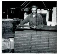
Workman applies adhesive to blocks of  $1\frac{1}{2}$ " FOAMGLAS precut to fit all the spandrel panel areas.
