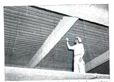
Underside of steel deck prior to application of Zonolite Direct-to-Steel Fireproofing. Oil, dirt removed for strong bond.
