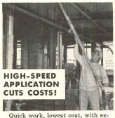
Quick work, lowest cost, with extension pipe applicator. At Onondaga County Bldg., undersides of steel floor were fireproofed throughout with Zonolite direct-to-steel fireproofing.
