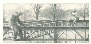
Steel Erection — V-LOK is an exclusive Macomber interlocking framing system that requires no on-the-job bolting, riveting or welding.
