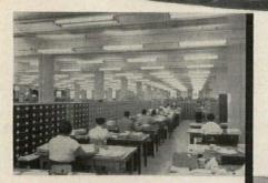
Original "Basic Unit" Rapid Start "Skyliner" bare lamp fixtures. Installed in 1952 when conversion into office building began, this was first large Rapid Start installation in the country. Original remodeling plans called for modernization of area in 1957. The ability to convert the "Basic Unit" to a modern, shielded fixture made it the perfect choice for this area.
