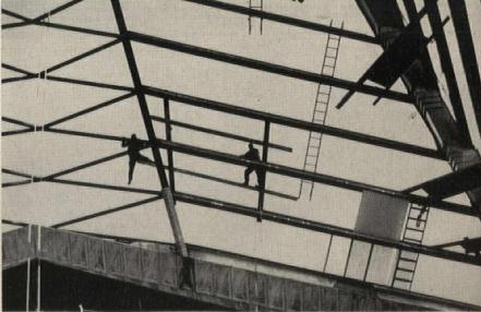
Above: non-vertical roof members are welded T beams which will also be faced with aluminum. Corrugated glass and plastic roofing panels may be seen on the lower right
