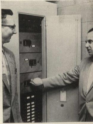
James Reil and Robert Lichtenthal check one of the two Westinghouse CDP panelboards which distribute 120 volts to the office machines from the Westinghouse 225-kva DT-3 dry-type transformer.
