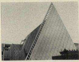
Intriguing design of aluminum checkerboard wall system combines aluminum glazing bars, mullions and operable vents with glass block and glass to provide an attractive pattern variation.
