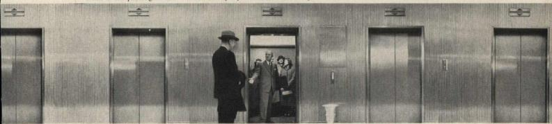
Here, Mr. Graves demonstrates how closing elevator doors will reopen instantly when a passenger crosses the threshold and breaks the electronic Traffic Sentinel beam which controls the door mechanism.
