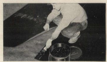
COMPARE the ease and speed of providing a permanent installation "PM" may be laid directly over the tamped grade or fill . . efficiently sealed with Sealtight Catalytic (non-setting) Asphalt, thereby providing a monolithic vapor seal with mechanically sealed joints, that will expand and contract with the concrete slab above, without breaking the bond.
