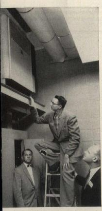
Robert Lichtenthal, James A. Reil, Ferguson Electric Construction Co., Electrical Contractors, and Charles Hansen discuss quietness and space-saving features which permit installation of Westinghouse 225-kva DT-3 dry-type transformer near office machines to which it supplies 120-v power.
