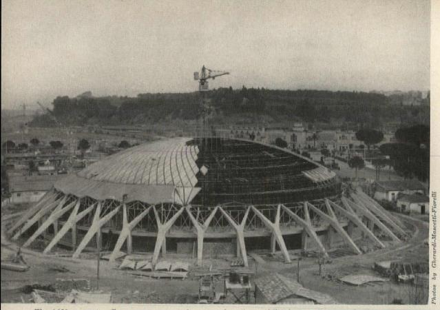
The 1620 precast coffers were supported on annular rings while the membrane and ribs were poured
