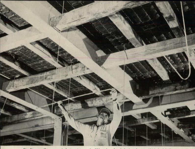
Steeltex easily spans six-foot centers on the fifth and sixth floor addition to Henry Ford Hospital in Detroit where it is supported by temporary shoring during pouring and curing. Bar mats provide reinforcing while Steeltex
