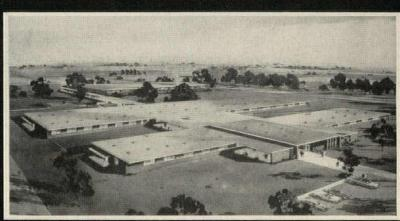
WARD BUILDING FOR MEXIA STATE SCHOOL, Mexia, Texas. Architect-Engineers: Thomas, Jameson & Merrill, Dallas. General Contractor: Eitze-Kitchen Construction Co., Dallas. Roof Applicator: Rodco Roofing Co., Waco. Zonolite Concrete over corrugated metal deck.
