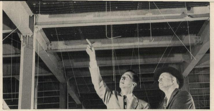
Steeltex gives clean, neat appearance underneath slab after shoring is removed. Pittsburgh Steel Products Salesman Russ Nutter shows A. M. Downes, field engineer for sub-contractor, Whitacre Engineering, how easily ceiling hangers were placed through Steeltex paper, thereby eliminating costly drilling of individual holes when wooden forms are used. Architect: Albert Kahn Associated Architects and Engineers of Detroit.
