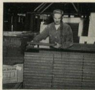
Workman applies adhesive to blocks of 1½" FOAMGLAS precut to fit all the spandrel panel areas.
