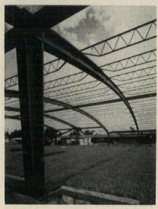
Detail of arch-to-column connection at outer end of 89 ft span shows carry-through of 1% in, plate. Wide flange beams welded to arches and columns serve as lateral bracing; bar joists between them are welded to brackets on arch webs. Columns are bolted to footings at base, connected by tierods.
