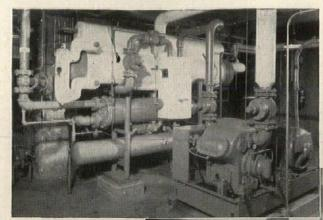
This Vilter air conditioning plant consists of a Freon shell and tube water chiller, shell and tube condenser, iquid receiver and a six-cylinder Freon VMC compressor, all installed in the Southwestern Bell Telephone Co., Olathe, Kansas,
