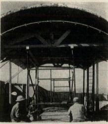
Forms are lowered from completed vaults with hand cranks, laid aside for re-use
