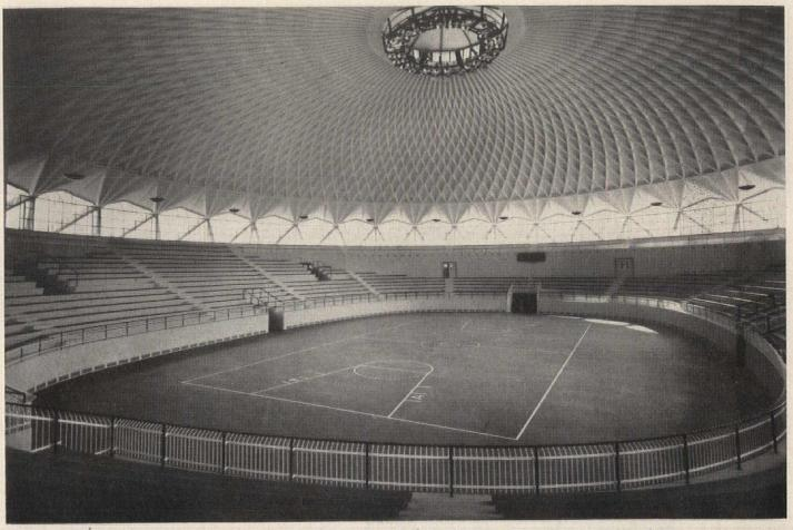
The elegantly patterned dome appears to float due to the continuous ring of glazing at is support points
