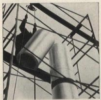
Installing this stack is quick and easy. Three-joot sections are simply cemented atop one another with acidproof cement.
