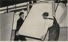
2 Gasketed panel is set onto aluminum frame
