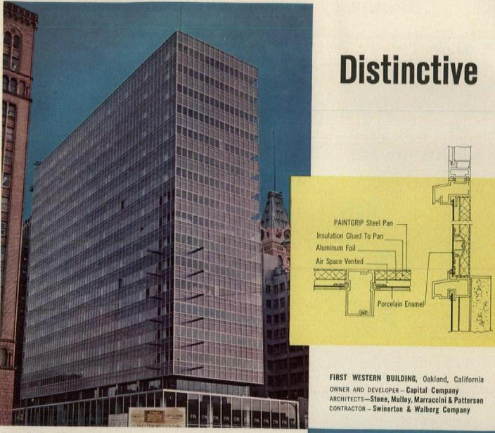
Floor-to-floor, modular porcelain enamel curtain wall units were entirely prefabricated, permitting quick erection from inside the building. CURTAIN WALLS-Kawneer Company, Berkeley, California PORCELAIN ENAMEL-Ferro Enameling Company, Oakland, California
