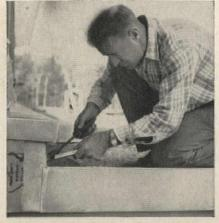
No Problems. Good workmanship is as easy to achieve in corrosion-resisting Monel alloy as it is in any other roofing metal. Neither fabrication nor installation of Monel sheet metal roofing requires special tools or techniques.
