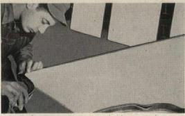
1 One-piece neoprene gasket is snapped over glass panel edges
