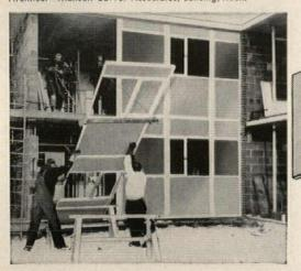
These lightweight panels incorporate Haskelite's own Polyester Resin impregnated fiberglass cloth faces, bonded to cement asbestos interbands, and a foamed polystyrene core.
