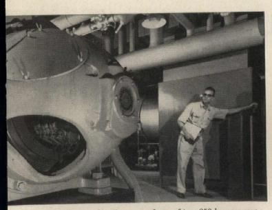
Operator is adjusting rpm of one of two 250-hp compressor motors. On-off switch is on column at right and motor control components are in large enclosed cabinet.
