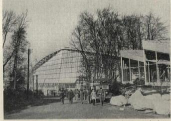
French Pavilion (Guillaume Gillet, architect) is composed of two hyperbolic paraboloids with surfaces forced by steel cable mesh; at the meeting point of these two forms a 200-ft-high mast will be constructed in the shape of an inverted V: supports, once intended to be confined to pilings under point of V, are also being put at two points at rear, a change forced by soil conditions.
