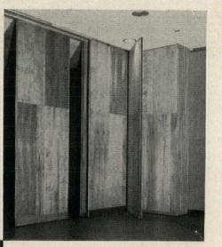
Units fold compactly to one side at the Dinkler-Plaza. Possible variations allow complete concealment of wall in special packets.
