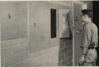
Westinghouse Type NLAB Quicklag® breaker lighting panelboards. A total of 42 lighting panelboards and 10 power distribution panelboards are installed in the hospital.
