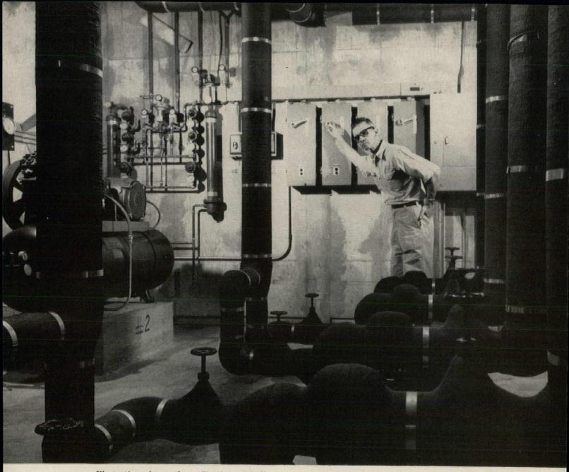
Illustration shows the utilization of individual Westinghouse motor controls. The four vacuum pumps in the foreground are individually controlled by the motor controls being operated in the background.
