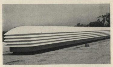
This lowered roof-top polyester-reinforced housing spans an area more than 100 feet long and protects 36 ventilating fans which exhaust chemical fumes from the building's laboratories. Resistant to corrosive fumes, this monitor section is actually an integral part of a laboratory fume-venting system that makes use of molded reinforced plenums and ducts.
