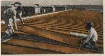
**Permanently Tight Joints.** No other commercial metal solders like copper. Cross joints in the roof pans at the crown are clinch locked, soldered. Ends of pans are pre-tinned.
