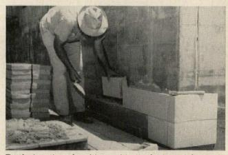
Tough, impact- and moisture-resistant polyester-coated concrete blocks are easy to lay up, provide handsome exterior or interior walls. The facing itself, a sand-resin slurry, is permanently bonded to the masonry unit. Color ranges are unlimited, particularly for interior uses where ultraviolet intensity is not a factor.
