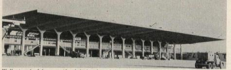
Wall at end of hangar (far left in photo below) indicates outset of hinged, canopy-type sliding doors which enclose two of six hangar positions, add 20 ft to their total usable depth
