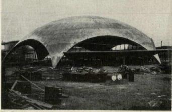
The Pavilion of the United Nations and its specialized agencies (Van Kuyck, architect) occupies an area of about 2650 sq yd. Its domed roof, with an interior completely of glass, rests on concealed columns. Auxiliary buildings on two sides of the main pavilion are interconnected by covered ramps. UN Pavilion is in International Section
