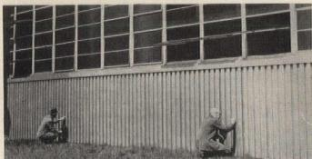
Typical wall section above was used to test methods of cleaning metal surfaces and applying protective coating. Method finally adopted was tested on panel at extreme right. Close-ups below show condition of original siding before and after lacquer application.
