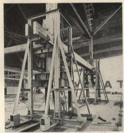
Traveler for nose hangar at Miami closely resembles that used for TWA hangar, but extra depth of corrugations made two-lift jacking necessary. Hydraulic jacks were used to lift and lower; sand jacks supported traveler between 6 ft lifts and during pour
