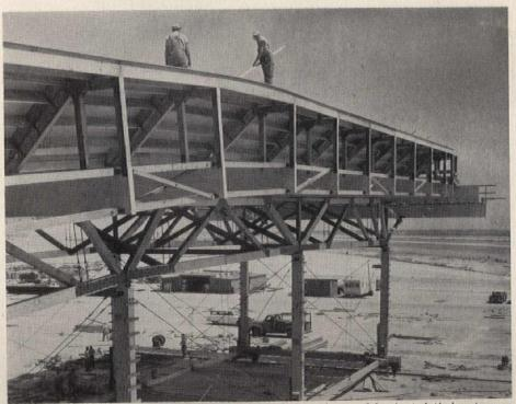
Similar hangar for TWA was formed using travelers made up of laminated timber trusses on eight posts braced by cross beams and steel rods. Hydraulic jacks at each column raise forms and lower them 6 ft to clear corrugations; sand jacks support them during pouring
