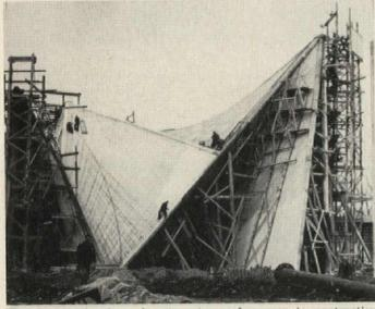
The photographs above show two stages of progress in construction of LeCorbusier's pavilion for the Philips Company, a Belgian manufacturer of electronics equipment. It is a system of two inclined surfaces which produces a volume of 141,600 cu ft from a surface area of only 5380 sq ft; there are no supplementary columns. Some 2000 concrete panels less than two in. thick form the surfaces; the
