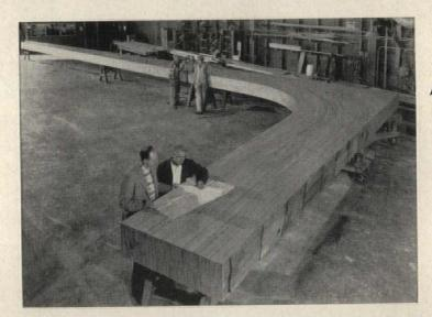
At Timber Structures, Inc. we call this swastika-like object the cat's whisker gauge. It is an important part of our quality control system. With it, frequent checks are made of the thickness of material being surfaced for lamination.
