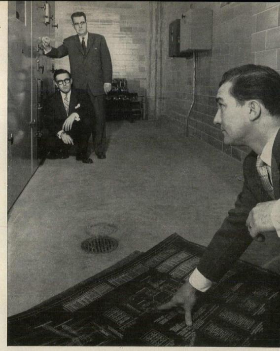
Contractor and engineers discuss metal-clad switchgear employing preferred-emergency incoming line transfer arrangement.
