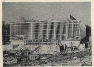
U.S.S.R. Pavilion—just across the street from the U.S. building was assembled of elements prefabricated in the Soviet Union and shipped to the site: the design was much affected by the Soviet plan to reconstruct the building in the U.S.S.R. as a permanent exhibition hall after the Fair is over. Architects: Alexandre Boretski, Urii Abramov, Victor Doubov and Anatoli Polanski.
