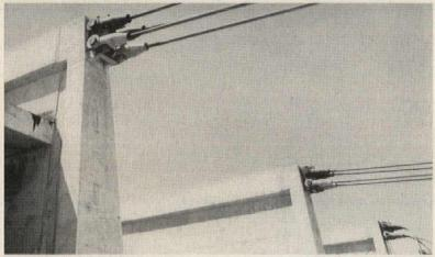
Outer ends of cables, with sockets attached, are drawn through sleeves in the valleys of the roof. Sixteen cables, 8 on each side, are tensioned at a time
