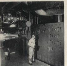
One of the two motor control centers with Type B wiring installed in hospital by Westinghouse. Each starter has 480-to 110-volt individual control transformer.
