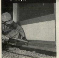
Sealing Around Mullion and Sill Joint in an aluminum-porcelain window wall.
