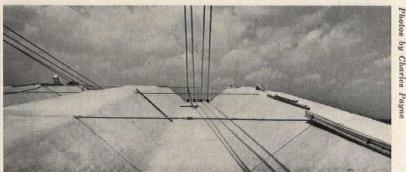
being built—one for National Airlines at Miami, the other for Mohawk Airlines at Utica, N. Y. (still in the early stages of construction—depart from the original in that their corrugated roofs are pure cantilevers. Shorter required spans made it possible to omit the suspension cables; nose pockets in the center section and canopy-type sliding hangar doors added enough depth to accommodate even large planes.
