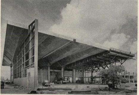
Giant "earthworks" shows scale of double span. Total hangar width is 270 ft; cantilevers extend 110 ft on each side of 50 ft center core, taper from 12 ft at roof to 3 ft at free end
