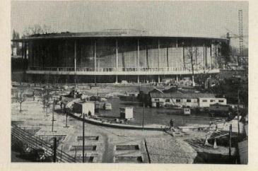
polyvinyl covering to resist wind loads with far less section than would be the case with conventional construction. Bicycle wheel roof of polyvinyl plastic fiberglass spans 300 ft (inner ring shown below is 60 ft in diameter and 24 ft deep), has gold-painted steel mesh suspended below it. Wall strips are white steel with gold rosettes, columns also gold-colored
