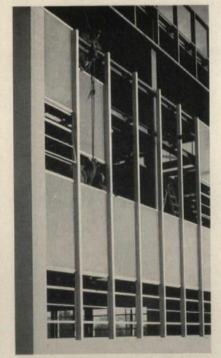
Lightweight (3 lbs. per sq. ft.) curtain wall panels are moved easily into place. Each unit is a weather-resistant plastic sandwich: 2-inch foamed styrene core between reinforced polyester plastic skins. Exterior and interior colors are built in. Because all components in the panel are insulators, heat loss is practically nonexistent.
