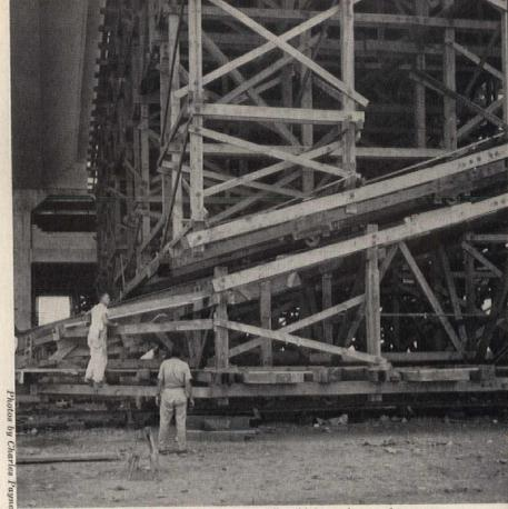
"Piggy-back" traveler for PAA hangar at Idlewild is made up of two sections of timber falsework with an inclined rail between. To lower forms, bottom wedge is allowed to slide forward under downward thrust of top section. Its primary advantage: lumber can be salvaged
