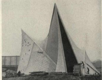
panels vary in shape but each covers an area of about 10.76 sq ft; they are held together with steel wires less than three tenths of an inch thick. An intricate and elaborate series of demonstrations has been designed for the interior: the effort being to show "light and sound integrally combined." No details on the demonstration have so far been made available.
