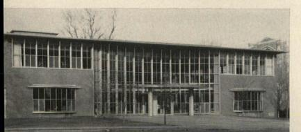
Close-up photo of front, curved glass wall which gives excellent light to interior—helped by the trim aluminum structural mullions which also contribute to the clean-lined design. Elliptical canopy is free standing . . . supporting columns are encased by aluminum extrusions.
