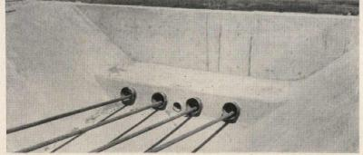
As cables tighten, slabs are lifted to final position. Lateral ties prevent sag before construction joints are poured between adjacent sections
