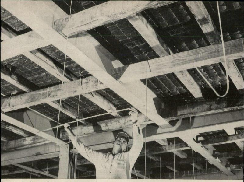
Steeltex easily spans six-foot centers on the fifth and sixth floor addition to Henry Ford Hospital in Detroit where it is supported by temporary shoring during pouring and curing. Bar mats provide reinforcing while Steeltex floor lath gives form to 3½ inch slab. Previously Steeltex was used on only 2- to 3-foot centers. The architect's decision to use Steeltex instead of wooden forms for six-foot spans was something new, but he soon saw it pay off as . . .
