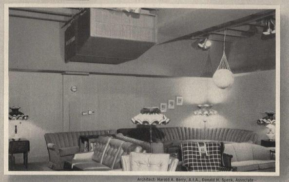
General Electric Ceiling-Mounted Units at the Dallas Home Furnishings Mart take no floor space -provide individual temperature control (heat and cool)-are metered for zone control of operating cost.
