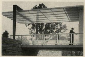
Translucent entrance canopy is a composite of 48 reinforced polyester sandwich panels: polyester skins covering a ½-inch honeycomb aluminum core. The canopy, fabricated to meet the minimum building code requirement of 30 lbs. per sq. ft. roof load, is fastened to the building at one end and is suspended at the other from a reinforced plastic bent of triangular cross section.
