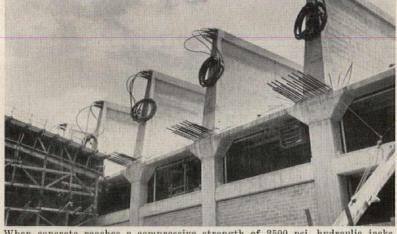
When concrete reaches a compressive strength of 2500 psi, hydraulic jacks are set up to tension the cables to an average stress of 176 kips in each
