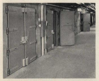
Test cells equipped with Jamison Sound Reduction Doors are in constant use. Jamison doors provide an average sound reduction of 50 decibels.
