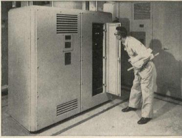
Transformer room view shows three of hospital's five Westinghouse dry-type self-contained power centers. 75-kva 208-volt wye to 120-volt delta ungrounded isolating power center is in the foreground, and two 225kva power centers are in the rear.
