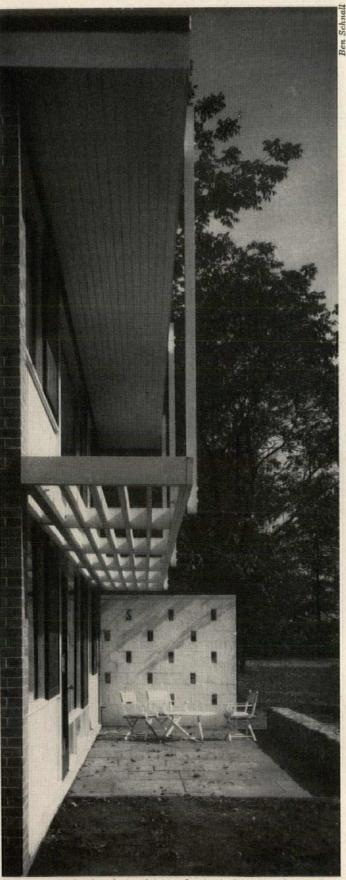
One can note, in the above picture of a typical terrace, how screenwalls of concrete block are employed to secure privacy. The block —which are painted light gray—are laid in a pleasing pattern of solids and voids that robs the screen of apparent heaviness. The louvered sunshade—in addition to serving its prime function—lends also a feeling of shelter to the terrace space.
