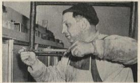
3 Pressure stop is screwed down to make a tight seal
