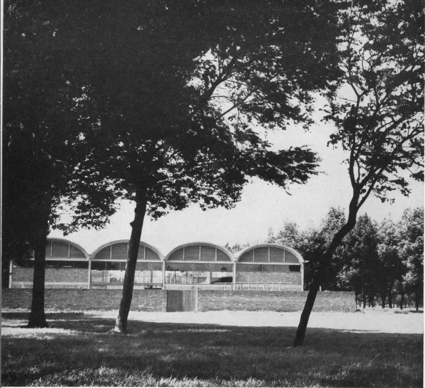
View from the north; wall encloses the experimental patio; thin-shell vaults of sprayed-on concrete roof the construction laboratory, making possible a room 66 by 120 ft without interior columns. Across page, air view of National University campus showing location of Housing Center
