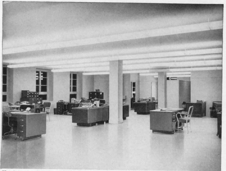
Here's an interior view showing a small part of the installation of Gold Seal Inlaid Linoleum. Actually, about 3½ acres of floor space are covered with this 1/8" burlap-backed "Veltone."
