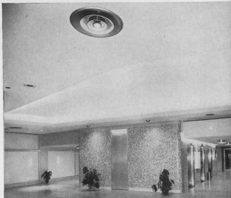
View of lobby showing Anemostat Air Diffusers
