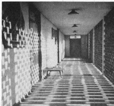
Bottom row, left to right: classroom corridor with sun-screen formed by an open brick grill; looking southwest in garden patio; conference room staff and students in round-table discussion; stairs to library mezzanine; library (mezzanine contains student lounge and space for additional researchers' offices)
