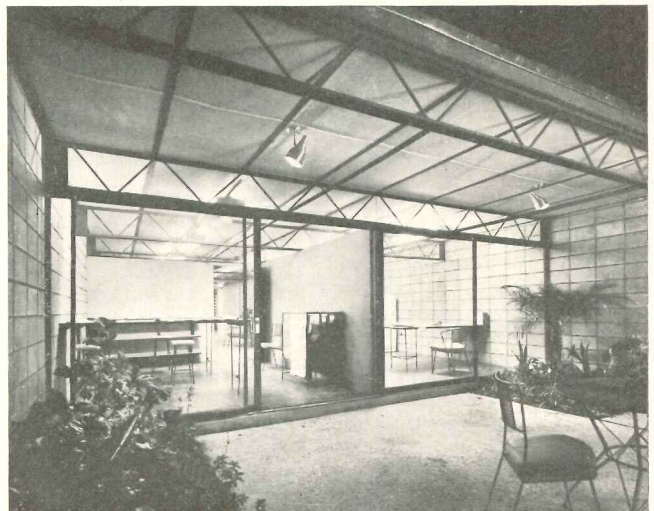
MERIT AWARD — Li Rocchi Building, Baton Rouge; Short & Murrell, architects. Rental offices for two tenants; cost $20,000
