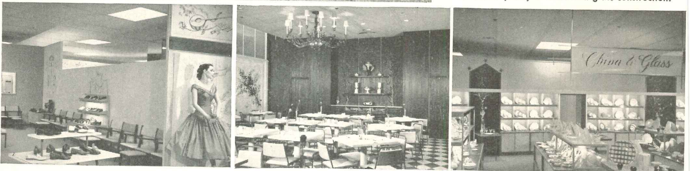
Modern lighting and automatic ceiling sprinklers give a clean, uncluttered appearance to various departments.
