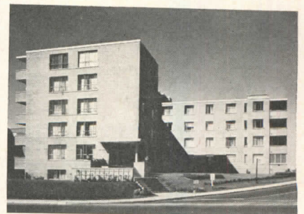
The Elmridge Apartments are some of many new units completed in Toronto's current apartment "boom"; Wilfred Shulman, architect
