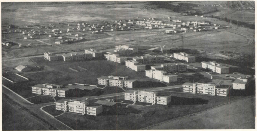
Spruce Cliff Apartments, at Calgary, Alta., were designed by architects Rule, Wynn and Rule, of Calgary
